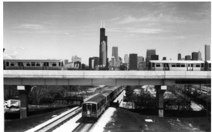
The Chicago Transit Authority operates all three types of rail fixed guideway--surface and elevated, shown here, and tunnel.
