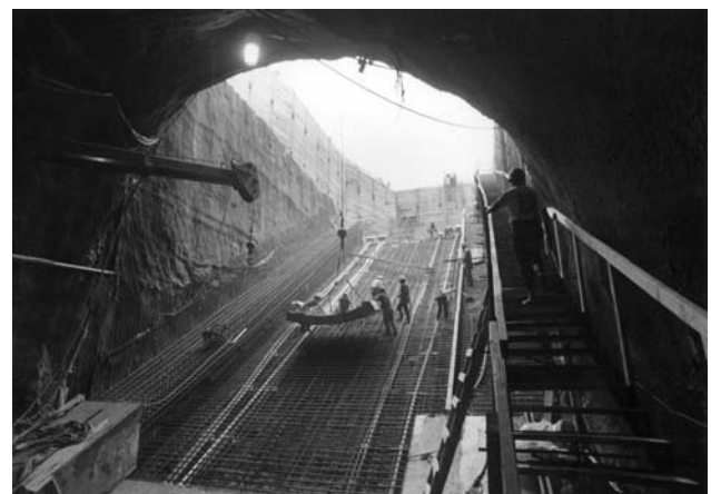
Major construction, such as this escalator for a Dallas Area Rapid Transit light rail line, pump millions of dollars into local economies.
