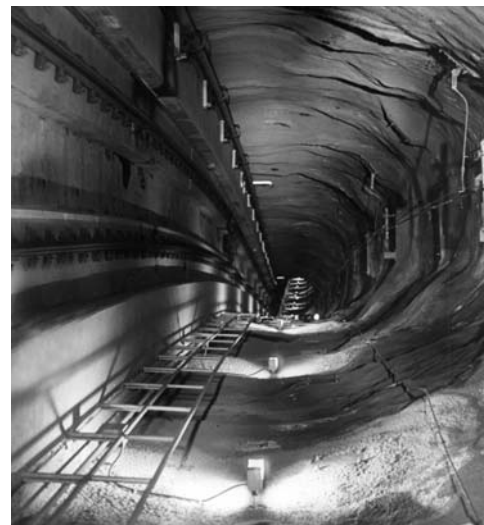
A Port Authority of Allegheny County light rail tunnel in Pittsburgh with walls left in a natural state. Some tunnels have finished walls and several tracks.
