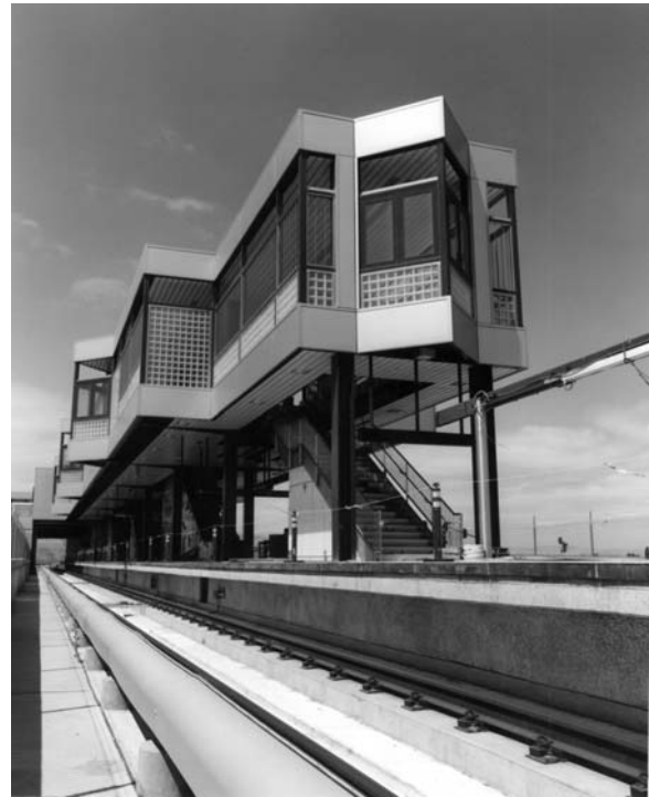
The San Francisco Bay Area Rapid Transit District Pittsburg/Bay Point Station shows not only high-platform design but also unique station architecture.
