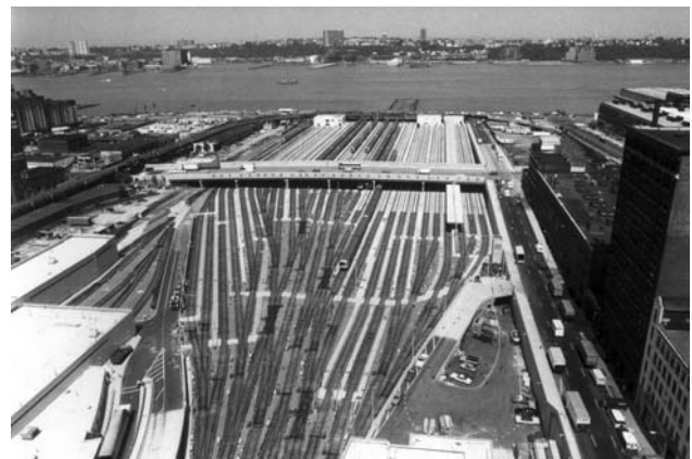
Among the capital projects constructed in recent years is this massive MTA Long Island Rail Road train storage yard west of Penn Station in New York City.
