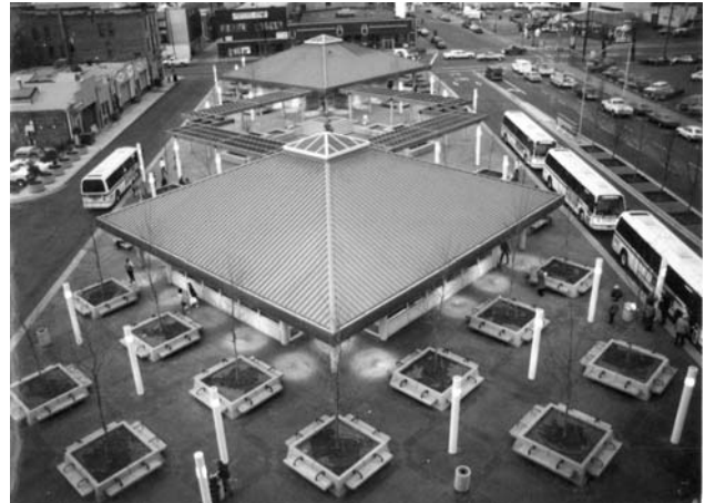
Many cities have built special transfer centers in their central business districts to make transferring between buses as easy as possible. Many also operate timed-transfer service, in which all routes converge on the center at the same time and depart simultaneously to minimize waiting time. This Regional Transportation Commission of Washoe County center is in Reno, Nevada.
