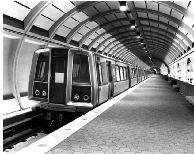
Modern rail station design minimizes crime by eliminating columns, dark corners, and other areas where criminals can lurk. This Washington Metropolitan Area Transit Authority heavy rail station illustrates such design.
