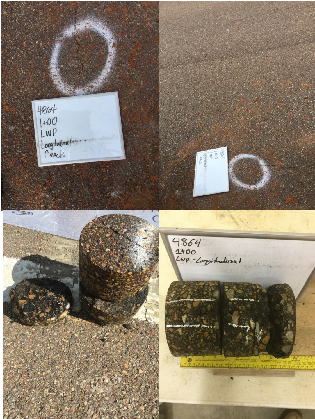
Figure 44: Pavement Surface and Core for Longitudinal Crack - Section 4864, Station 1+00
