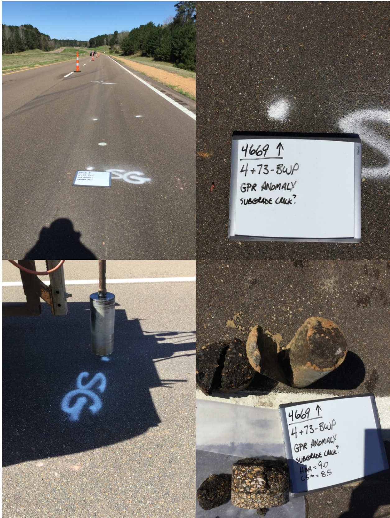
Figure 8: Core Cut at Station 4+73 – Section 4669
