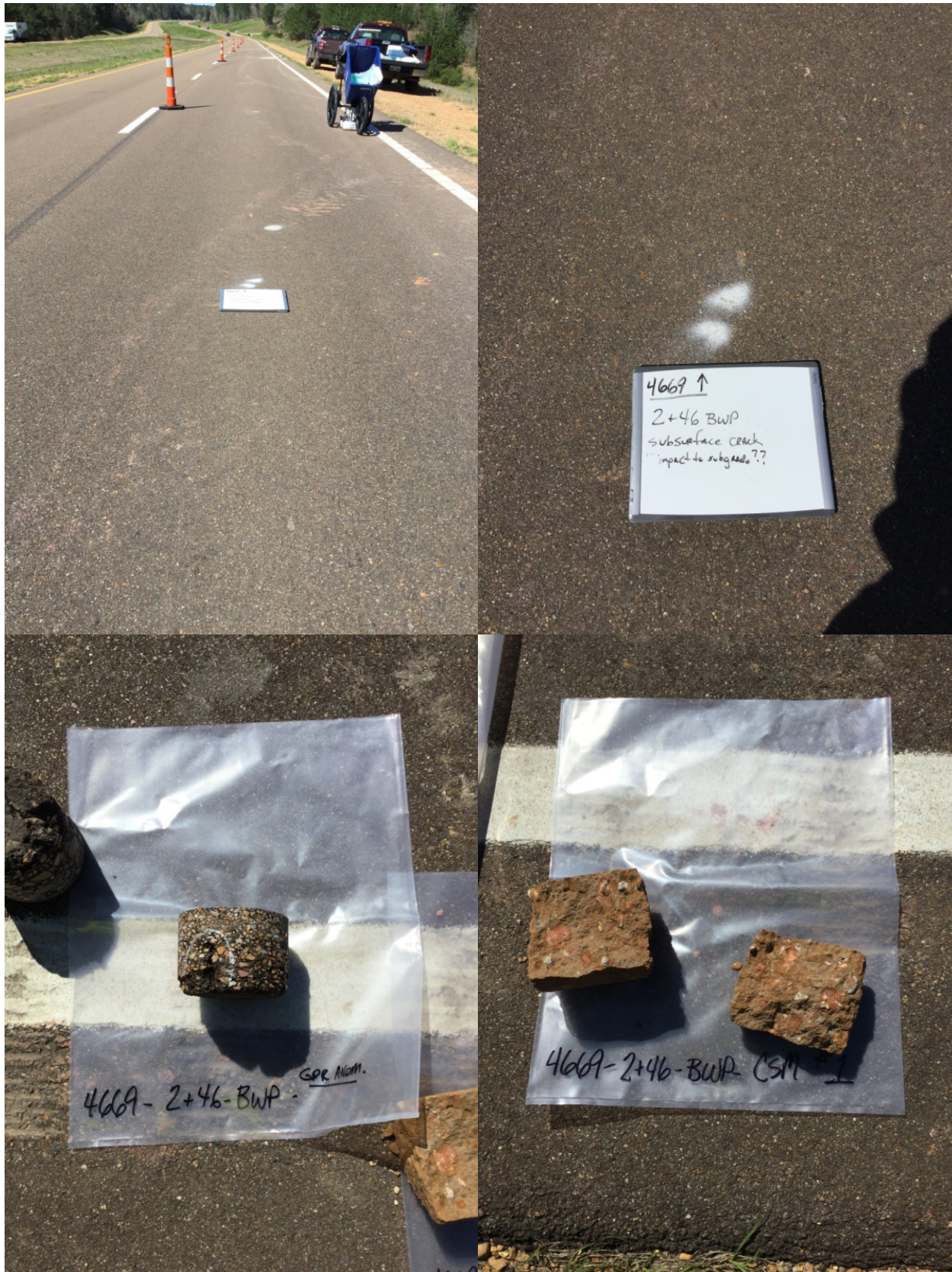
Figure 4: Core Cut at Station 2+46 - Section 4669
