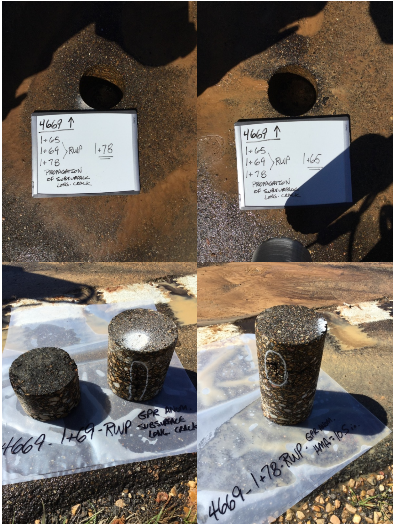
Figure 11: Cores Cut at Stations 1+69 and 1+78 – Section 4669
