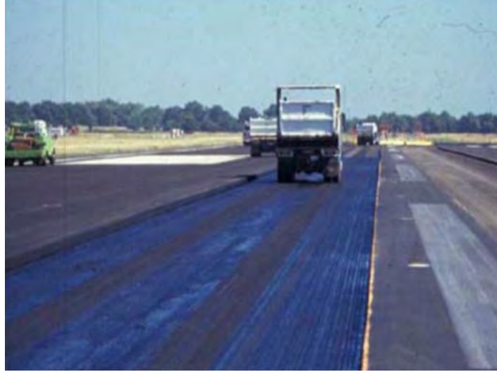
Figure 2.3: Tracking by haul truck during pavement construction (Mohammad et al. 2012).
