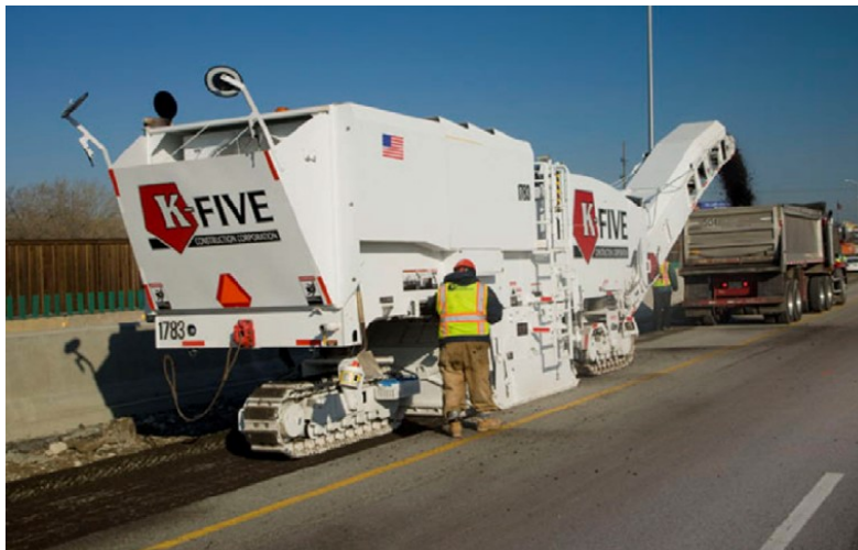
Figure 2.7: Pavement milling operations in the field (West 2010).
