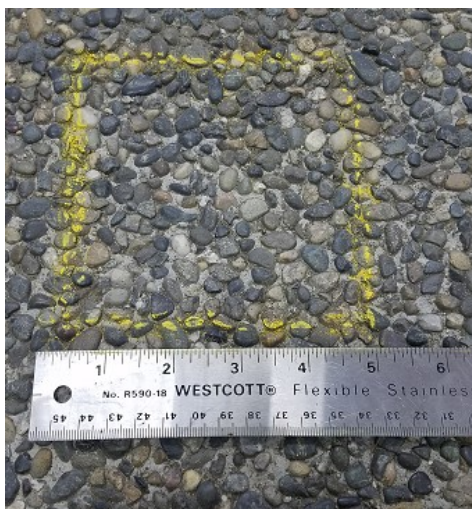
Figure 6.20: 5inch by 5inch square drawn on the pavement surface.
