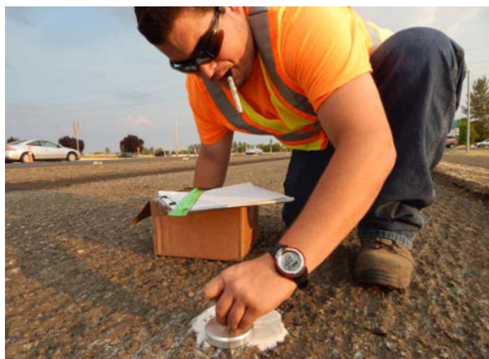
Figure 2.6: Sand patch testing on milled pavement surface (Coleri et al. 2017).
