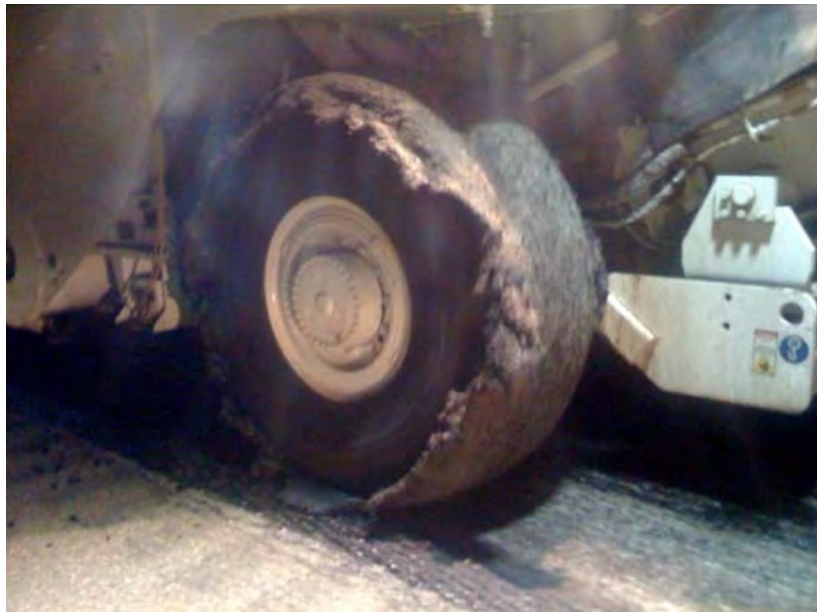
Figure 2.11: Tracking on paver wheels due to excess dust (Mohammad et al. 2012).
