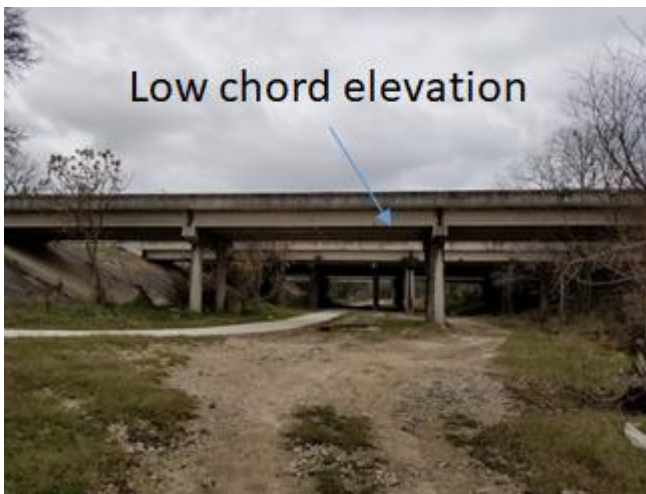
Figure 2-4 Low chord elevation (LCE)
