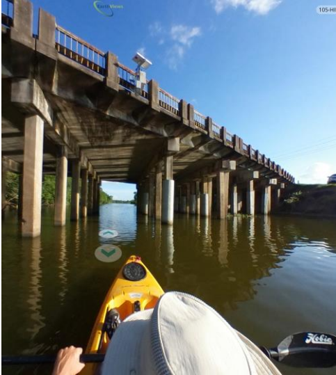
(a) Photography approaching bridge
