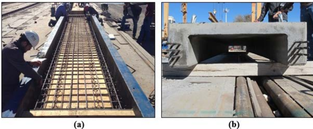
Figure 18. Girder H-PS-C-300-R-UO (a) reinforcement before casting and (b) after pre-stress transfer.
