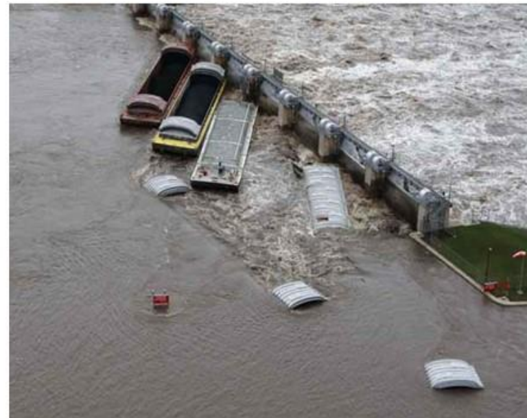
Source: ABC 7, Chicago – Flooding on Illinois River, Apr. 2013 http://cdn.abclocal.go.com/images/wls/cms_exf_2007/news/local/AP433827475512.jpg
