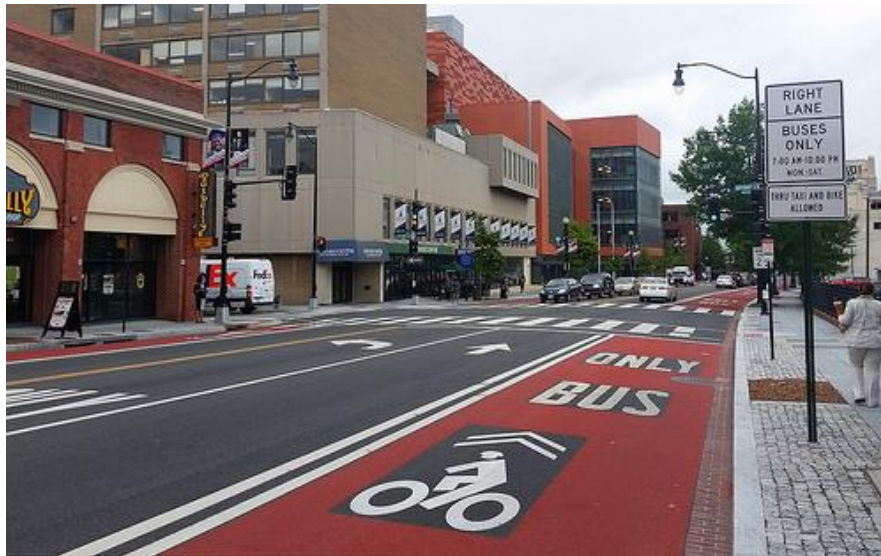
Figure 4. Marked bus lanes along Georgia Avenue NW 17
