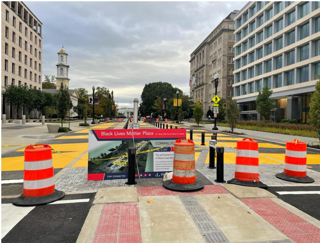
Figure 18. 16 th Street (NW)/Black Lives Matter Plaza Southbound Approach
