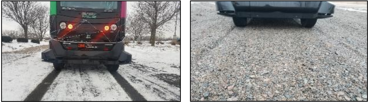
Figure 3-17 Observed Wheel Tracks
