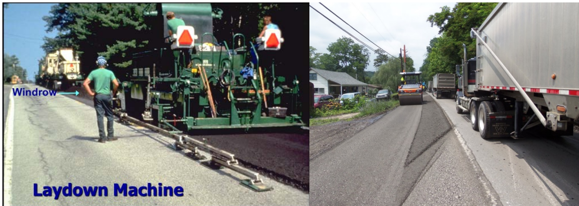
Figure 1.2. The CIR mix is picked up by the paver and roller compacted.
