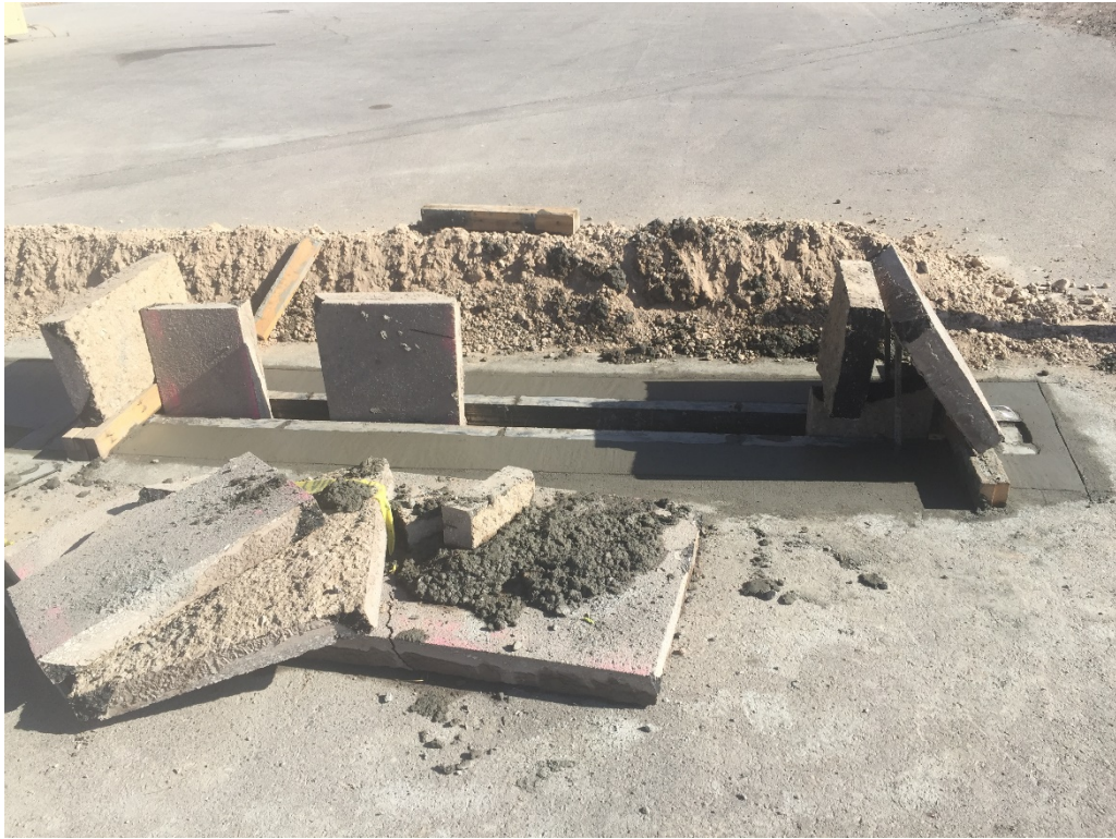
Figure 13. Installation in the Field of the Steel Housing for the Unit Box Beam and Roller Assembly.
