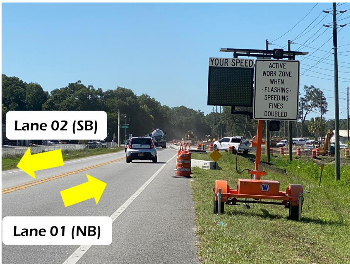
Figure 36. Field View for Phase 2A at US-98 and Trilby Rd
