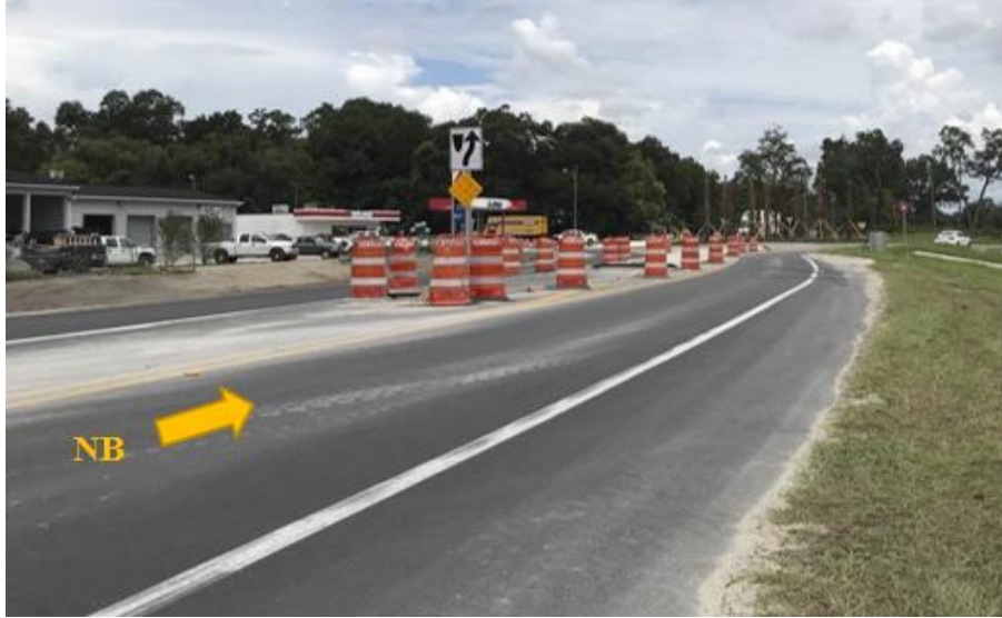
Figure 49. Field View of Phase 4B2 at US-98 and Trilby Rd
