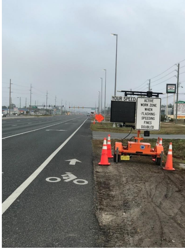
Figure 70. Field View of Construction Zone on US-19
