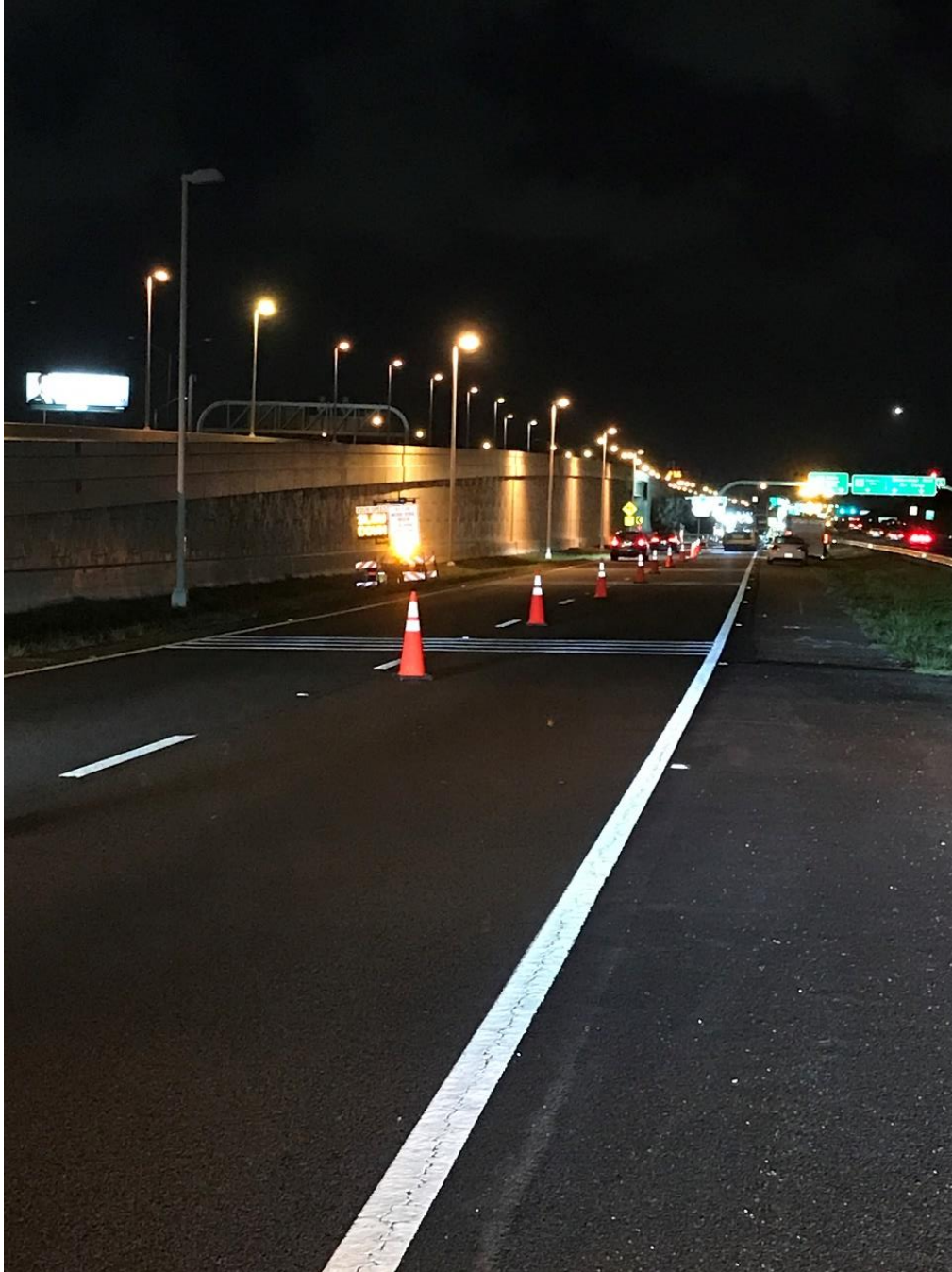
Figure 88. Outside Lane Closure at Site 8: Veterans Expressway
