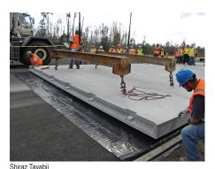
Figure 2. Placement of a precast panel
