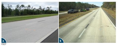
Figure 1. US 92 (FL-600) west of Daytona Beach, Florida: (a) condition of the existing jointed concrete pavement before overlay construction and (b) overlay condition as of February 2021
