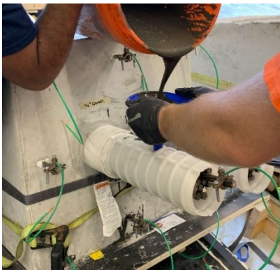
Figure 10. Photo. Grout placement using funnel through opening in top of duct. Copper grounding clamps with #10 AWG copper wire are attached to counter electrodes and tendon strand for electrical measurements.
