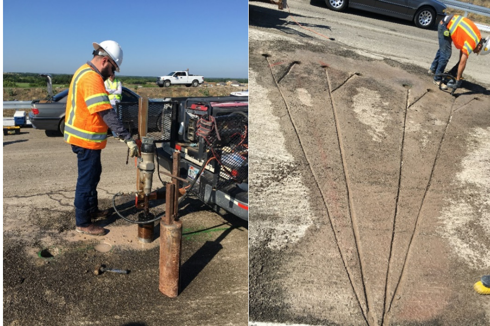
Figure 26. Coring and groove cut in the HMA base layer.
