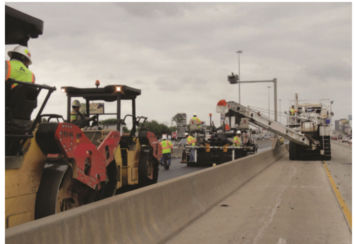
Construction of the Interstate 69 overlay system.
