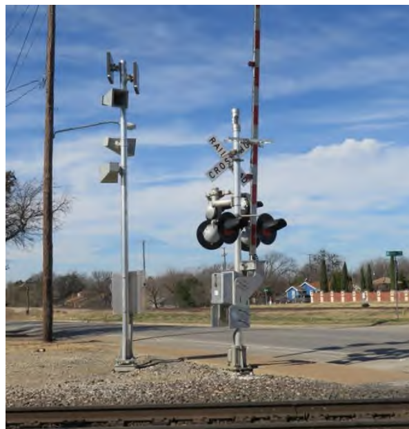
Figure 37 An example of a crossing bell. Source: U.S. DOT. (2019). Highway-Rail Crossing Handbook (Figure 26)
