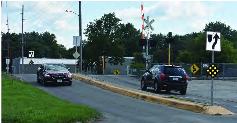
Figure 44 An example of two-quad gates with a raised median. Source: Donahey. (2019). Council Evaluating Railroad 'Quiet Zones'
