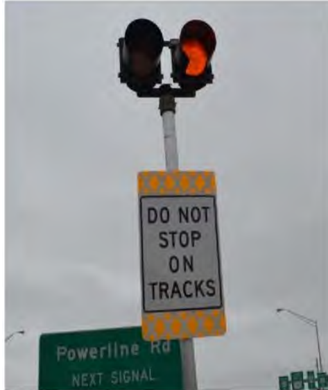
Figure 59 An example of a dynamic envelope zone modified signage.
