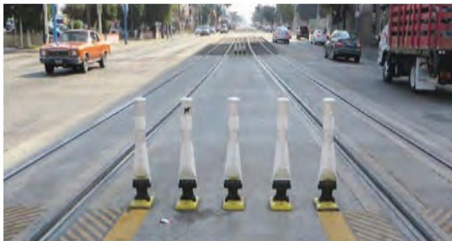
Figure 57 An example of bollards. Source: TCRP-175. (2015). Guidebook on Pedestrian Crossings of Public Transit Rail Services (Figure 158)
