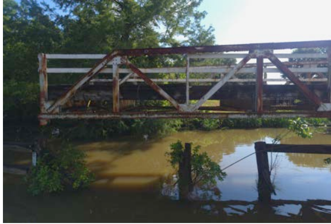
Figure 31. Upper view, bridge inspection, SW-side.
