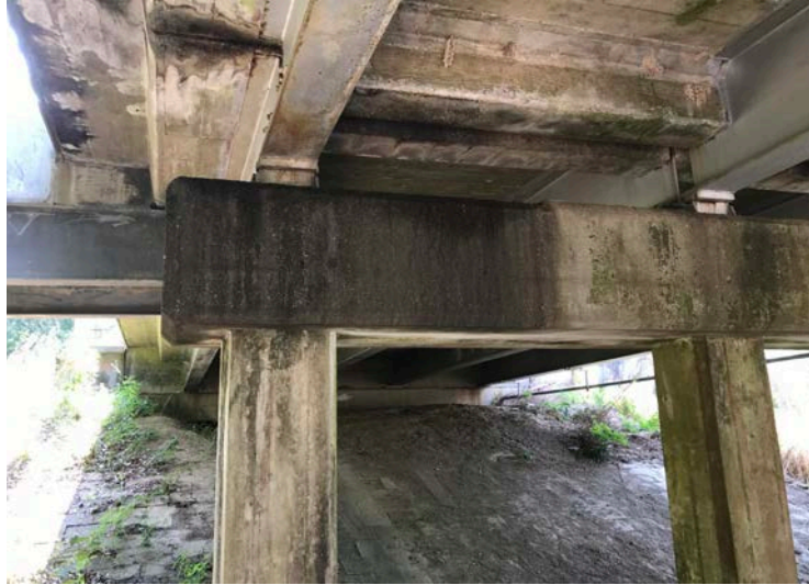
Figure 23. Shows tight space confinement beneath the deck of the sample bridge.
