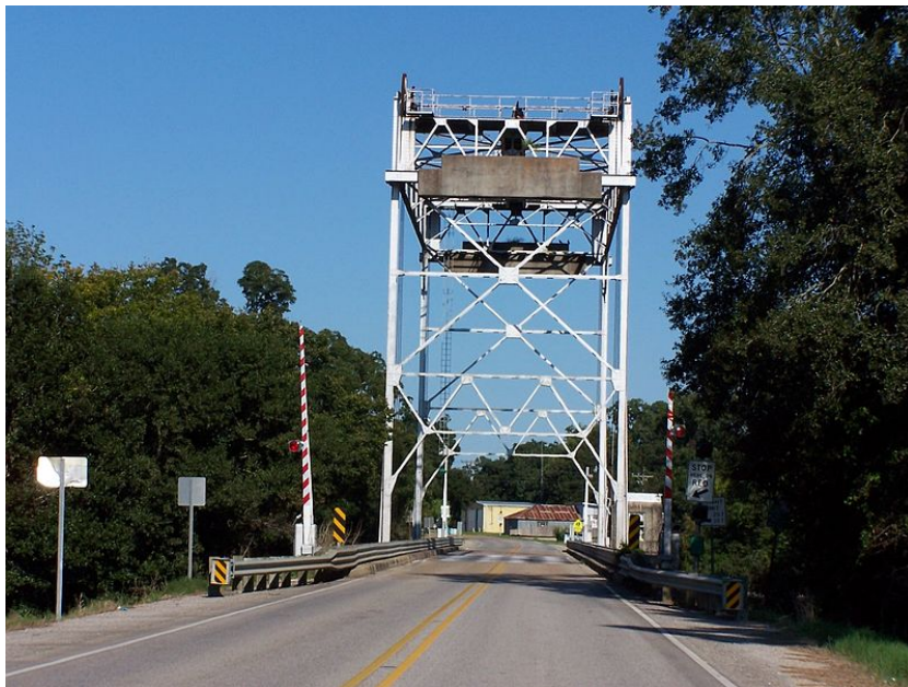
Figure 2. Vermilion River Bridge, Milton, LA – Example of a draw or lift bridge.
