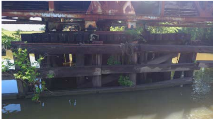
Figure 32. Lower view, bridge inspection, SW-side.
