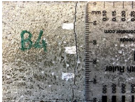
Figure 10 - Shrinkage cracking in an example test specimen.
