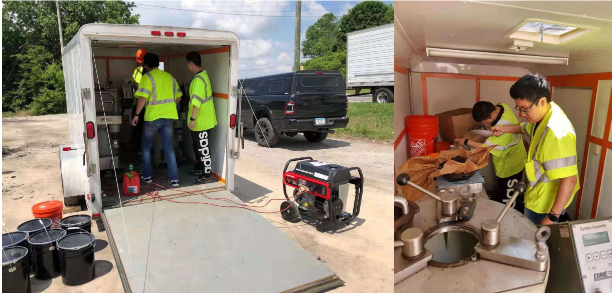
Figure A-2. UT mobile trailer and specimen compaction in the field.
