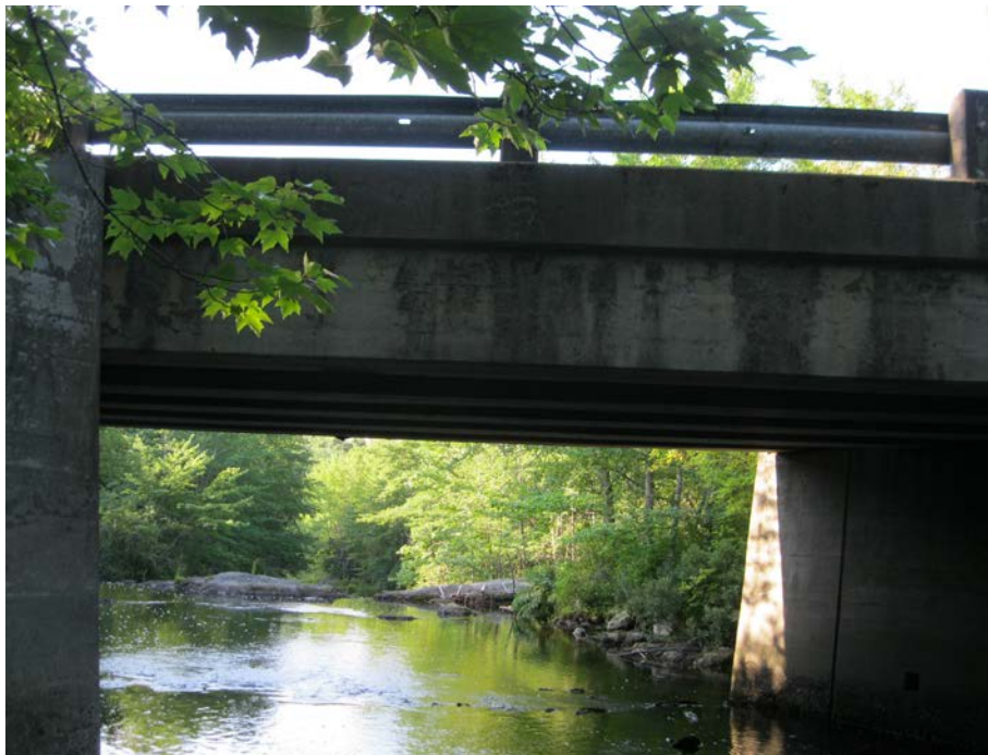
Figure 15: Bridge 3848 general condition
