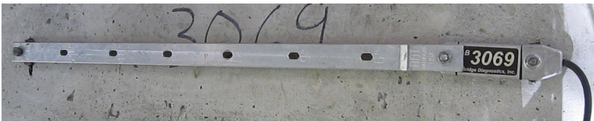
Figure 1: Typical strain sensor mounted under bridge, equipped with extension
