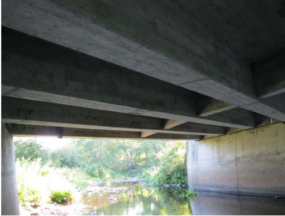
Figure 11: Bridge 5109 general condition
