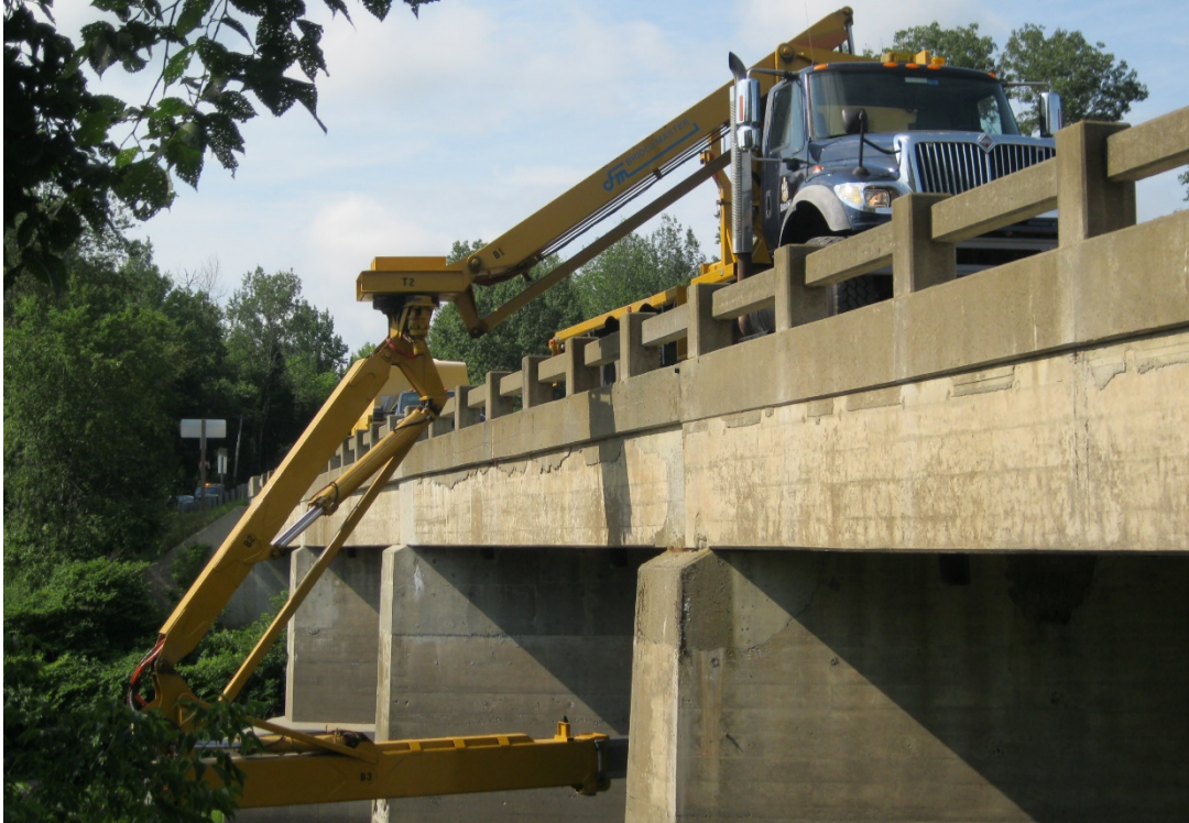
Figure 3: MainDOT UBIT used to install sensors
