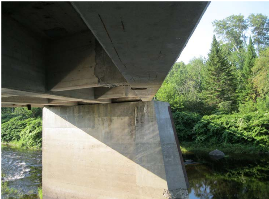
Figure 14: Bridge 2879 general condition
