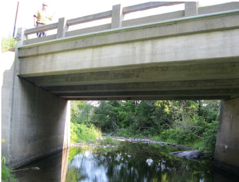
Figure 12: Bridge 2390 general condition
