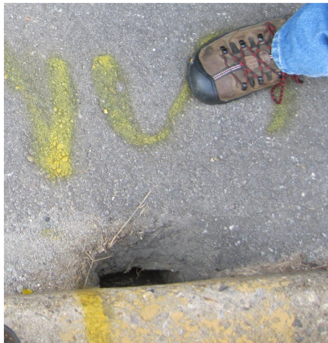
Figure 13: Thick asphalt overlay
