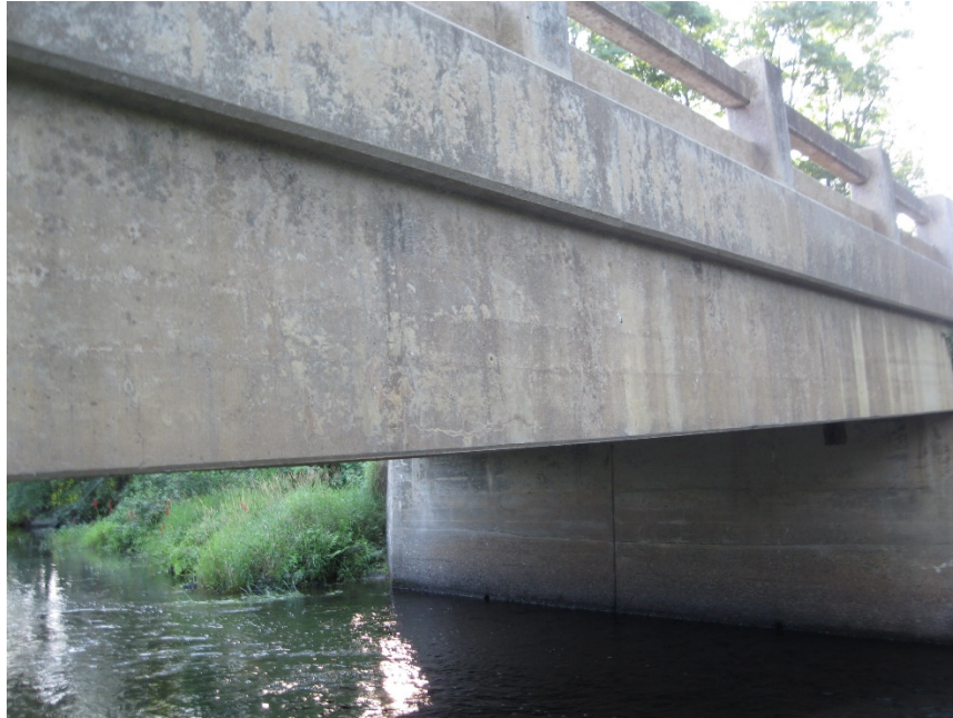
Figure 10: Bridge 5489 general condition
