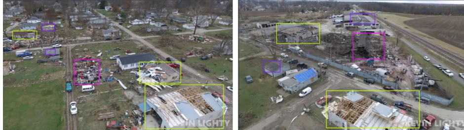
Figure 4-2 Example of annotated images. The blue, green, and purple bound boxes denote damages in slight, severe, and debris levels, respectively.
