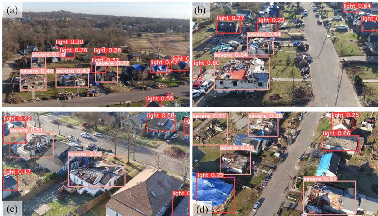
Figure 4-6 Detected Building Damages from Post-Tornado Structure Surveys.
