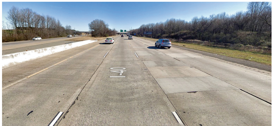
FHWA, Arkansas Division office
