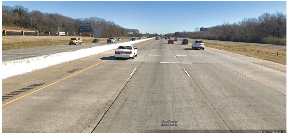
FHWA, Arkansas Division office
