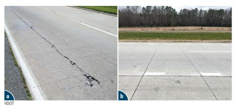
Figure 1. Westbound US 58 in Southampton County: (a) condition of the existing CRCP before overlay construction and (b) close-up view of the unbonded concrete overlay in January 2021
