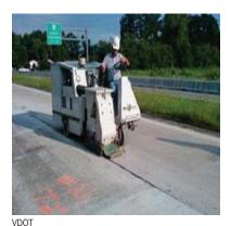
Figure 2. Shotblasting of existing CRCP surface
