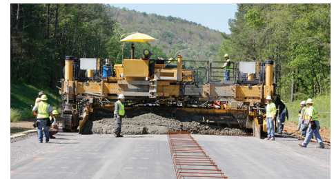
Figure 3. Concrete overlay placement in 2011
