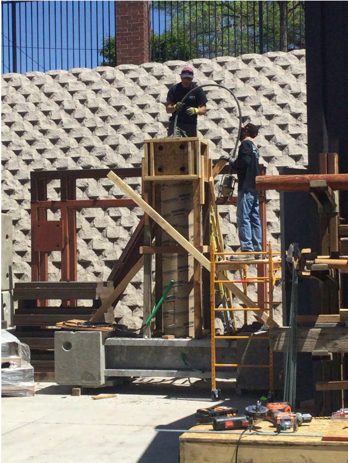
Figure 2.15 Vibrating of fresh cast concrete
