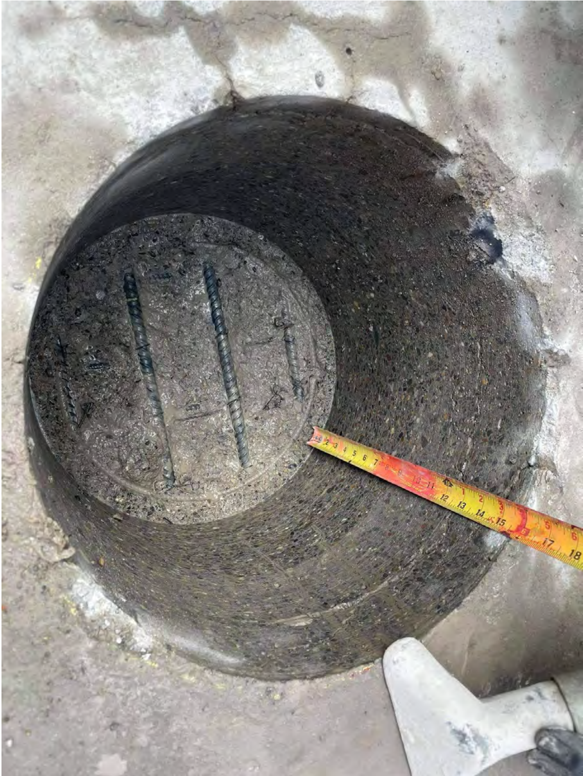
Figure 2.9 Joint pocket after coring
