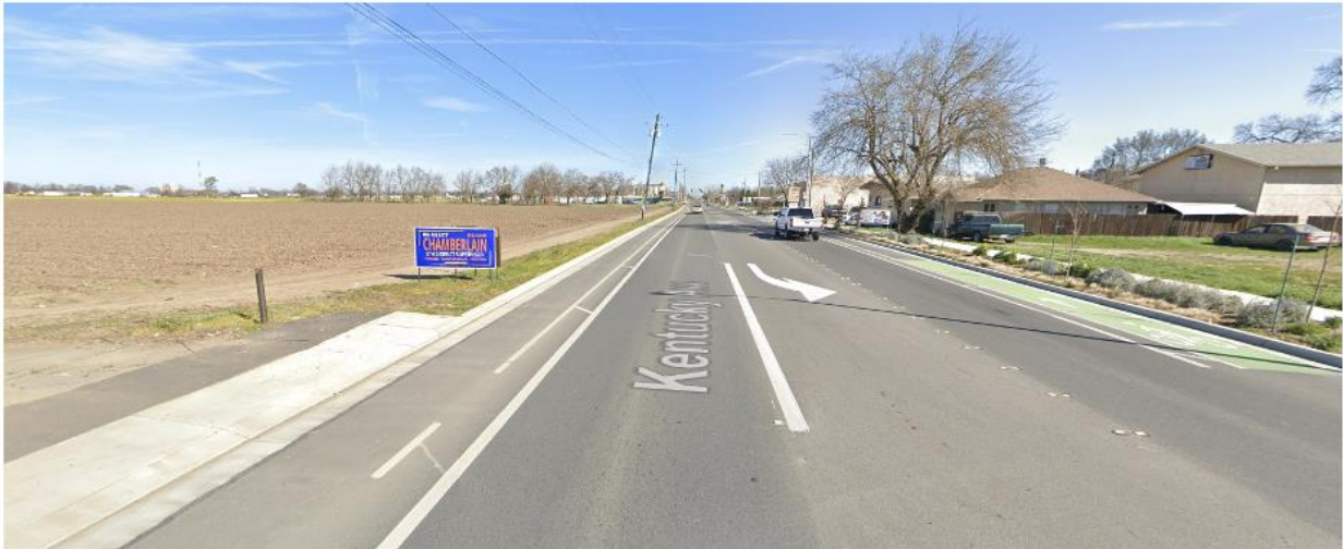
b) After adding the complete street features (Google Earth, 2020, Avenue has been updated with dedicated bike lanes and sidewalks)
