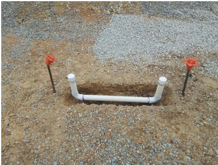
Figure 36. FFC placement pit site.
