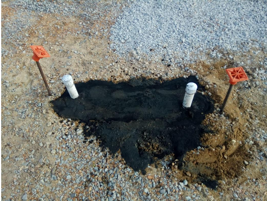
Figure 37. FFC mixture placing.
