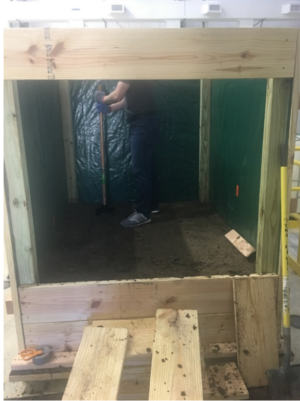
Figure 26. Compaction of soil at corners.
