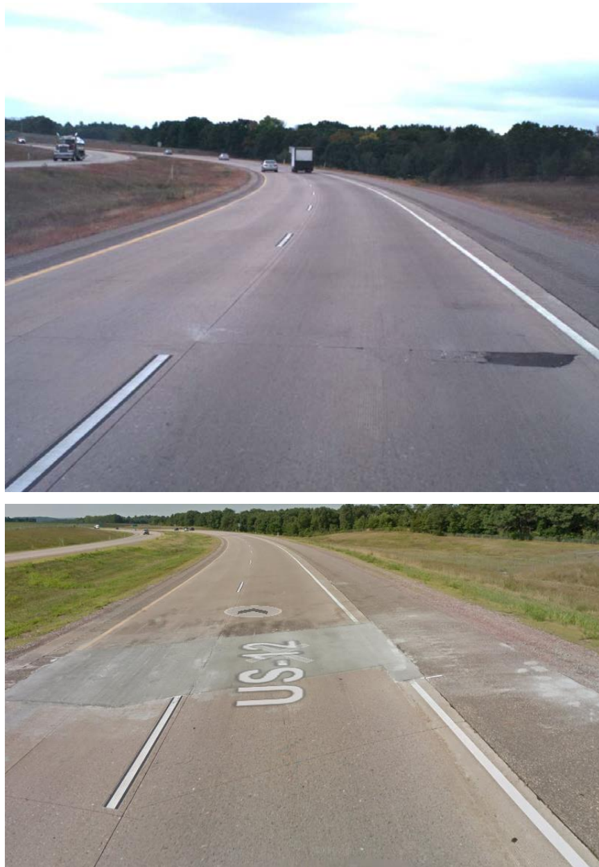
Figure 14. October 2017 Google Earth® images of U.S. 12 prior to buckling showing spalls and asphalt patching (top). July 2018 Google Earth® image of the same joint following buckling (bottom).
