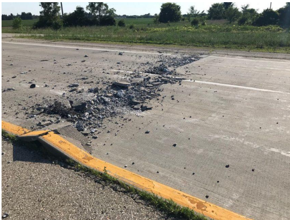
Figure 1. Blowup on Hwy 14 in Rock county (Courtesy: Rock County Sheriff's Office).
