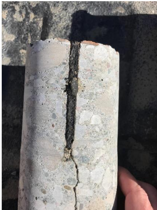
Figure 69. Core at the joint filled with sealant (MTO 2018).
