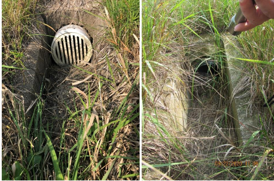
U.S. 29 WB in Chippewa Co., Site # 3 (left), I-39 SB in Columbia Co., site # 4 (right)
