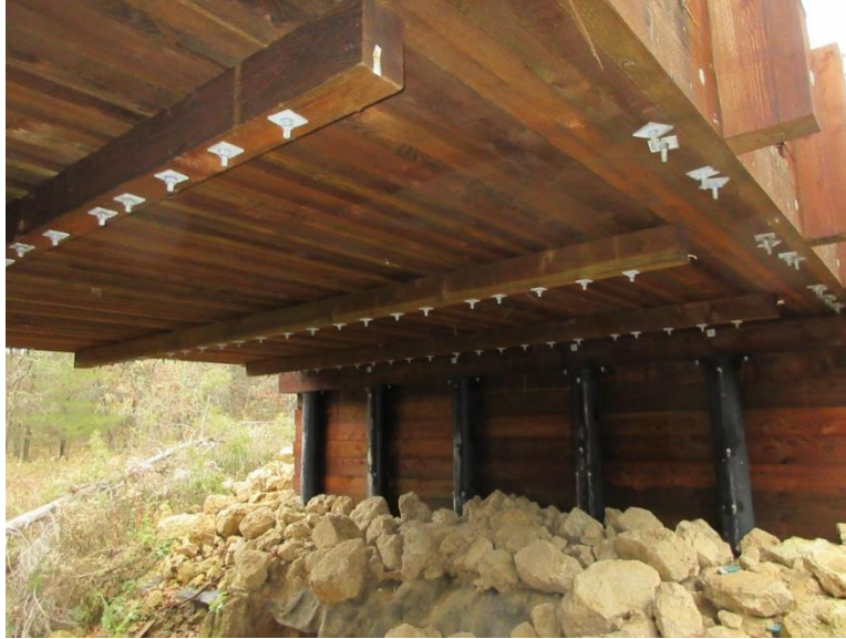
Figure 4-48 Monroe County Bridge B410315 Spreader Beams
