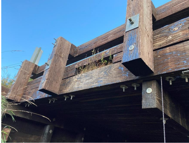
Figure 4-55 Vegetation in Curb Gutters (Barron Co. B030174)
