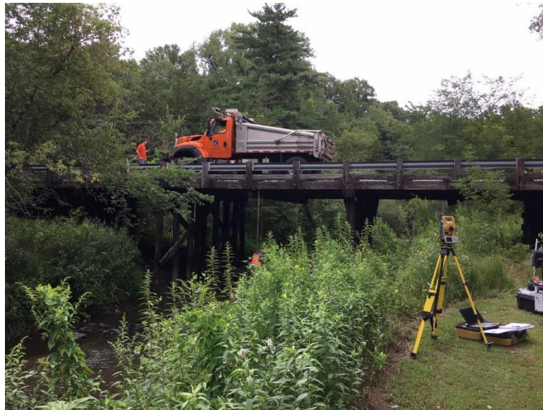
Figure 4-15 Truck parked at position of maximum strain response for survey data collection
