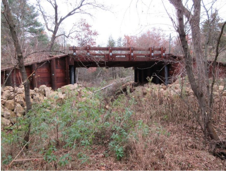
Figure 4-42 Monroe County Bridge B410315
