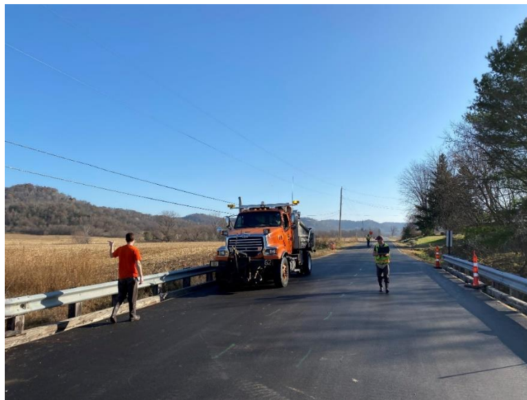
Figure 4-13 Load truck crossing the bridge
