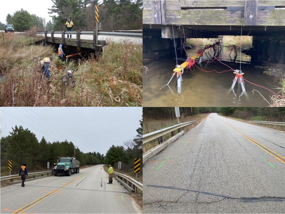
Figure A. 8 Bridge photos for P410953
