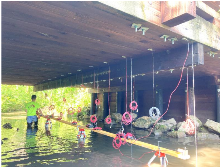
Figure 4-49 Sauk County Bridge B560224 Spreader Beam
