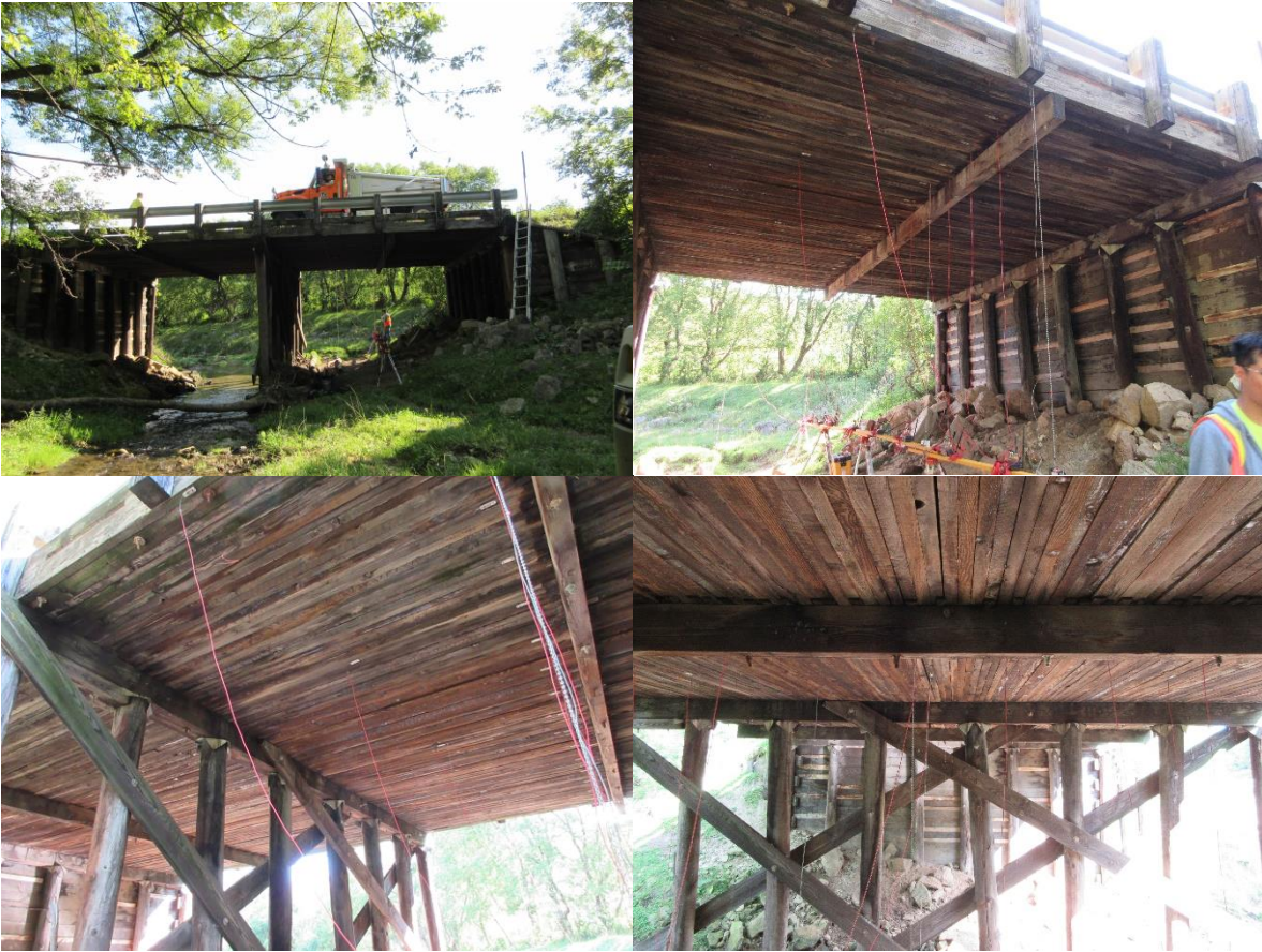
Figure A. 5 Bridge photos for P320110
