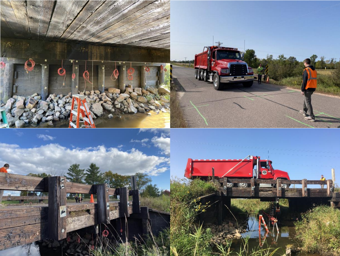
Figure A. 1 Bridge photos for B030174
