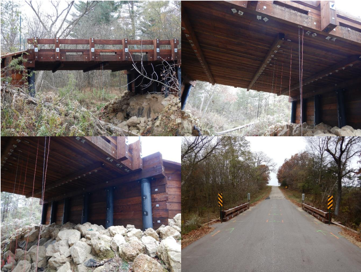
Figure A. 9 Bridge photos for B410315
