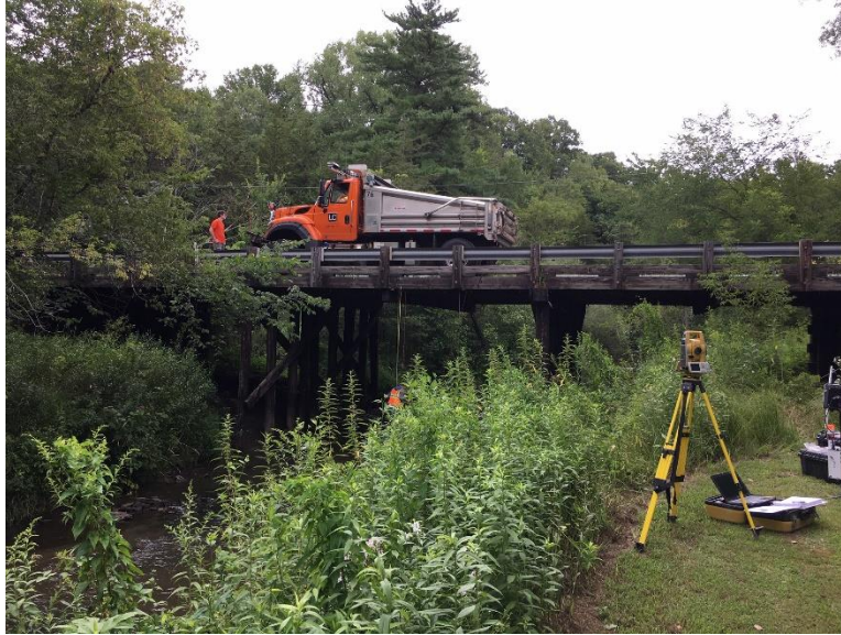
Figure 7-2 Deflection data collected via total station
