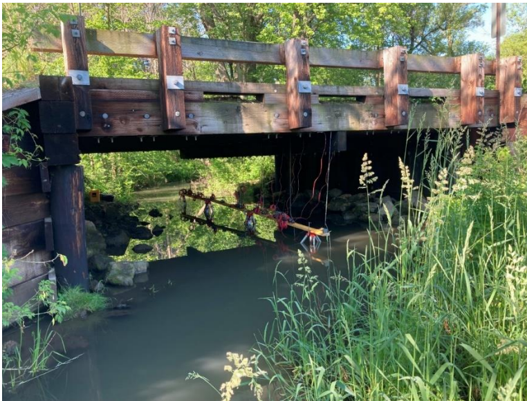
Figure 4-43 Sauk County Bridge B560224
