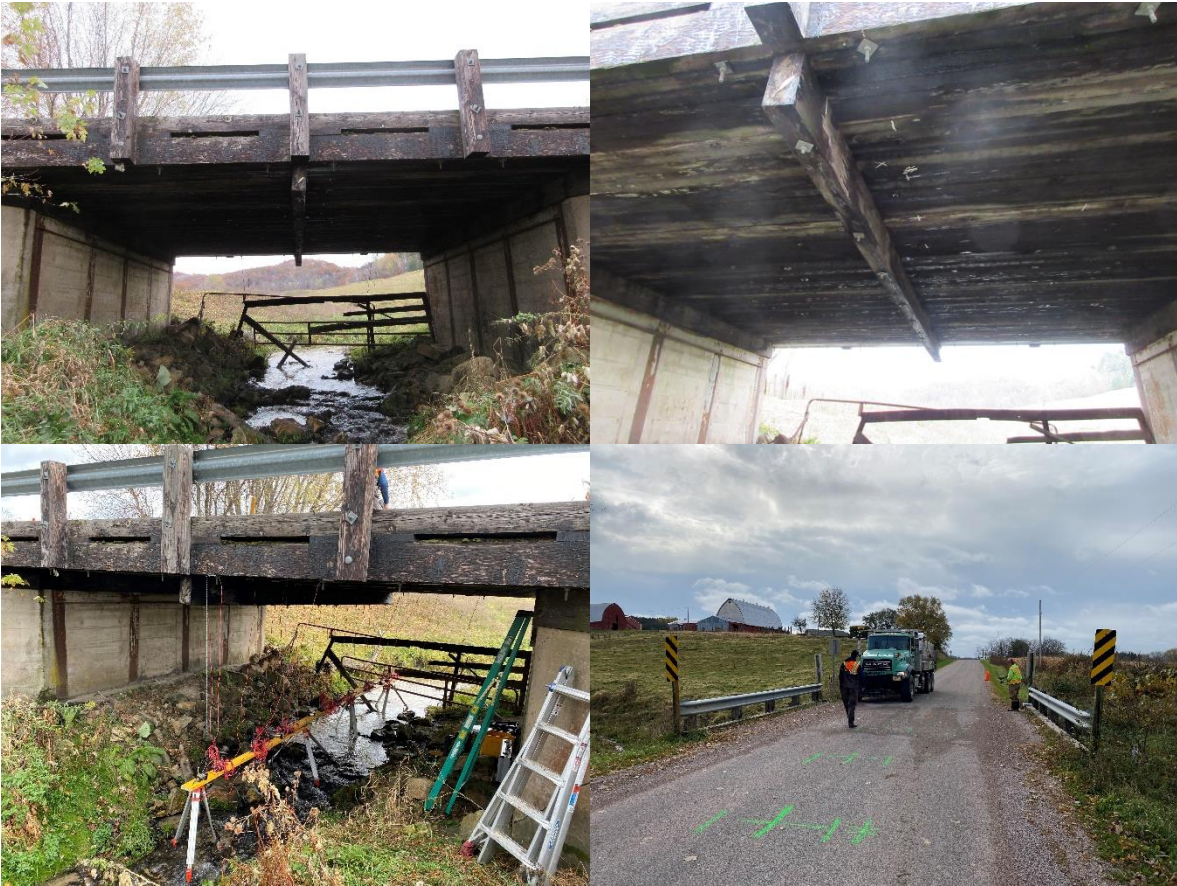
Figure A. 7 Bridge photos for P410923
