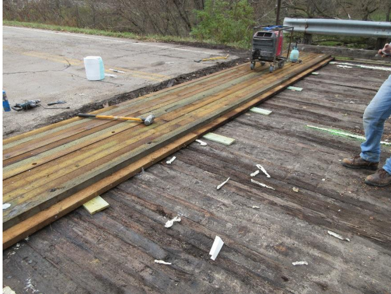
Figure 4-35 Transverse Timber Slab Retrofit under Construction
