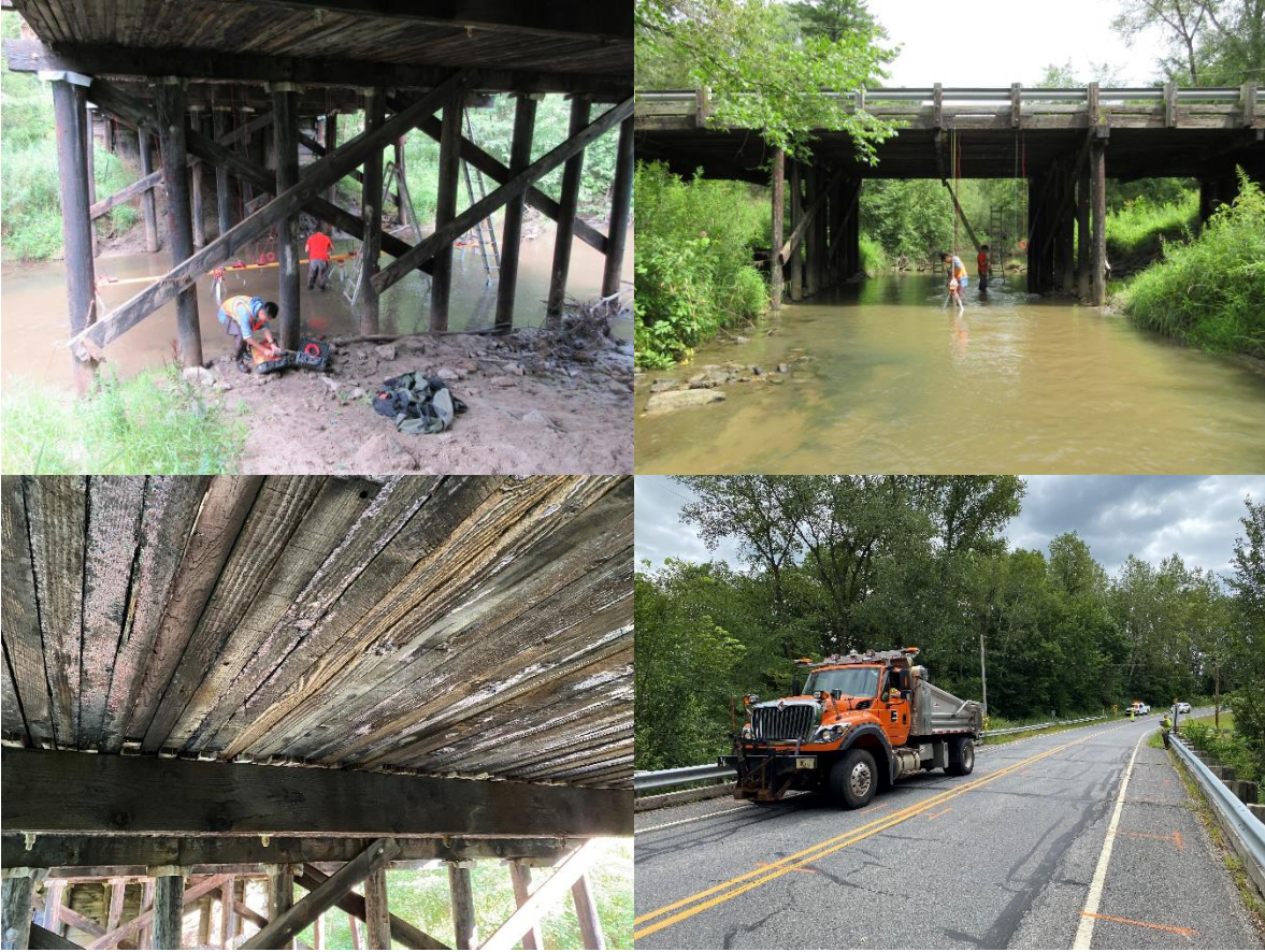
Figure A. 4 Bridge photos for P320083
