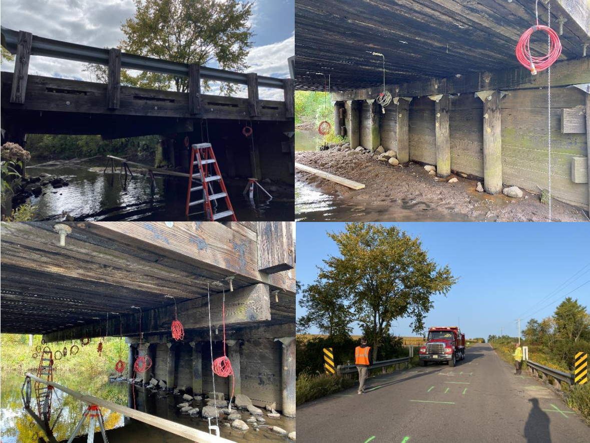
Figure A. 2 Bridge photos for P320079
