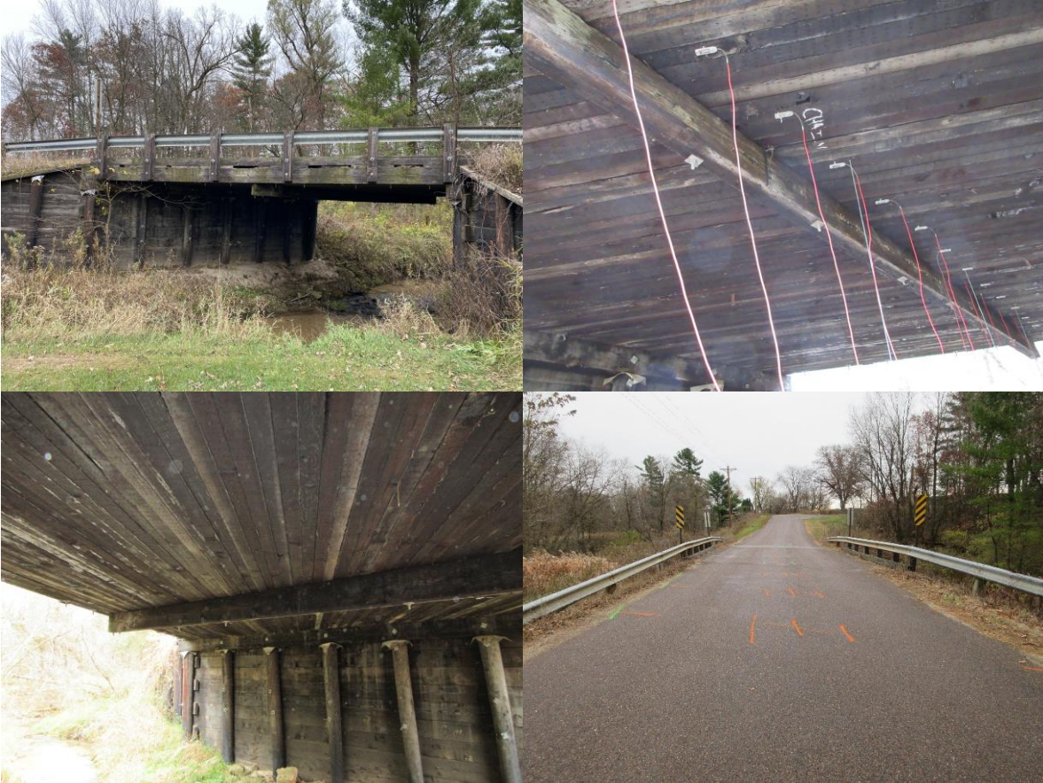
Figure A. 6 Bridge photos for P410140
