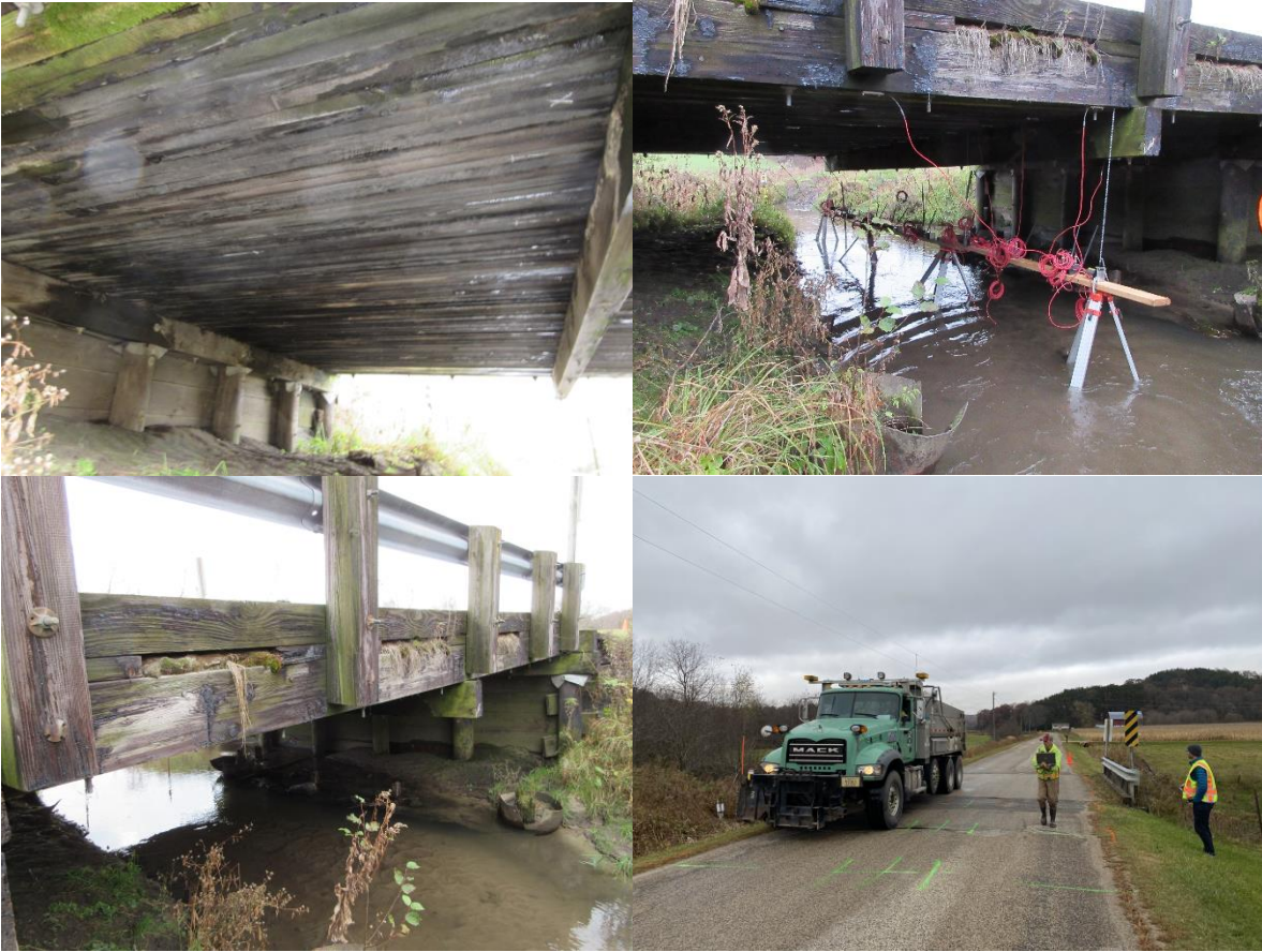
Figure A. 10 Bridge photos for P410948
