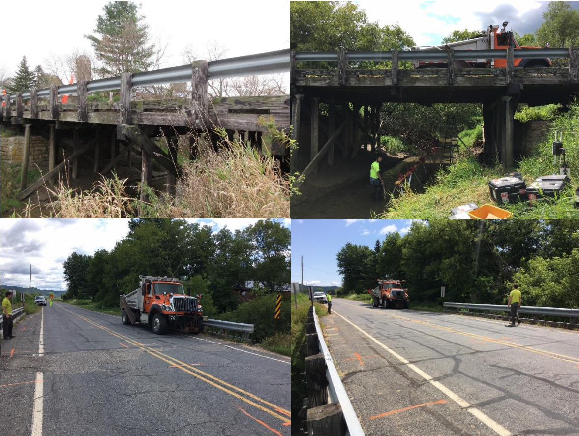
Figure A. 3 Bridge photos for P320064
