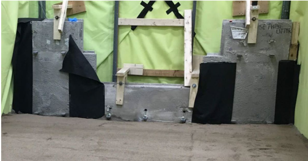
Figure 3-5. View from inside of facility displaying geotextile used to cover gaps between adjacent panels.
