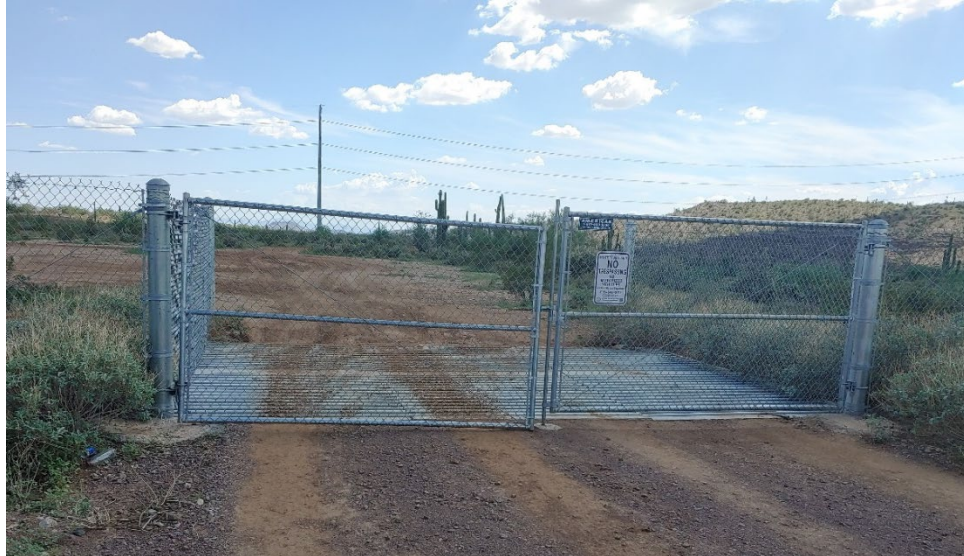
Figure 77. Gate Modified with Signage, a Crossing Guard, Wing Fence Tied in Within the Vault Ledge, and Spans of Chain-Link Flanking Fence on Both Sides of Driveway to Deter Trespassing
