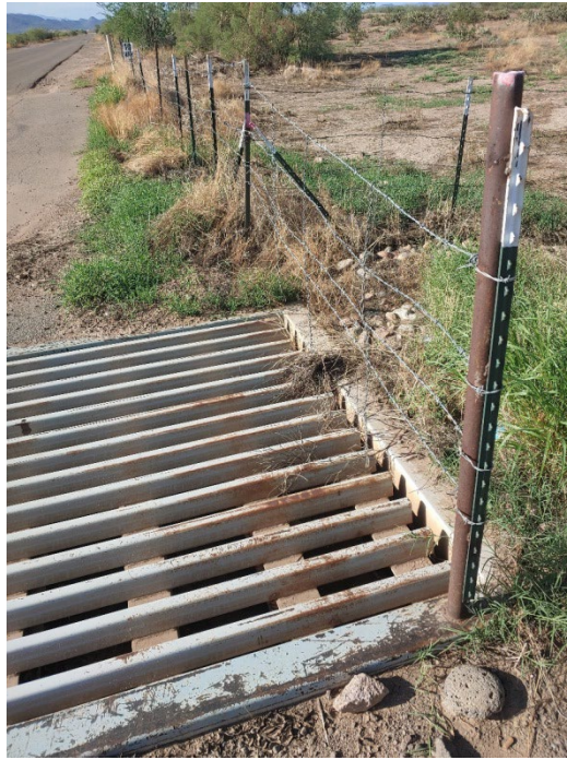
Figure 72. Wing Fence at a Crossing Guard Tie-In
