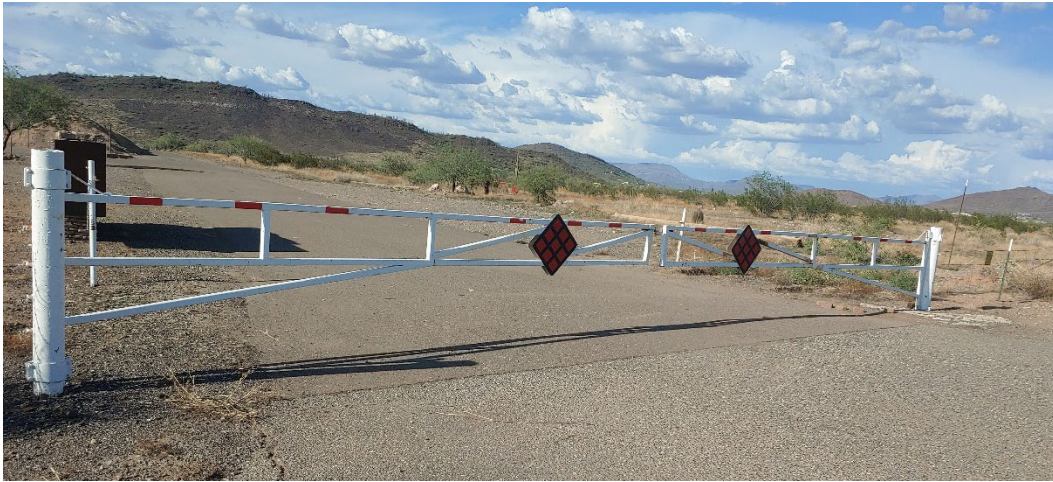
Figure 64. Single-Arm Gate with a Gap Greater Than 24 Inches Beneath the Bottom Bar
