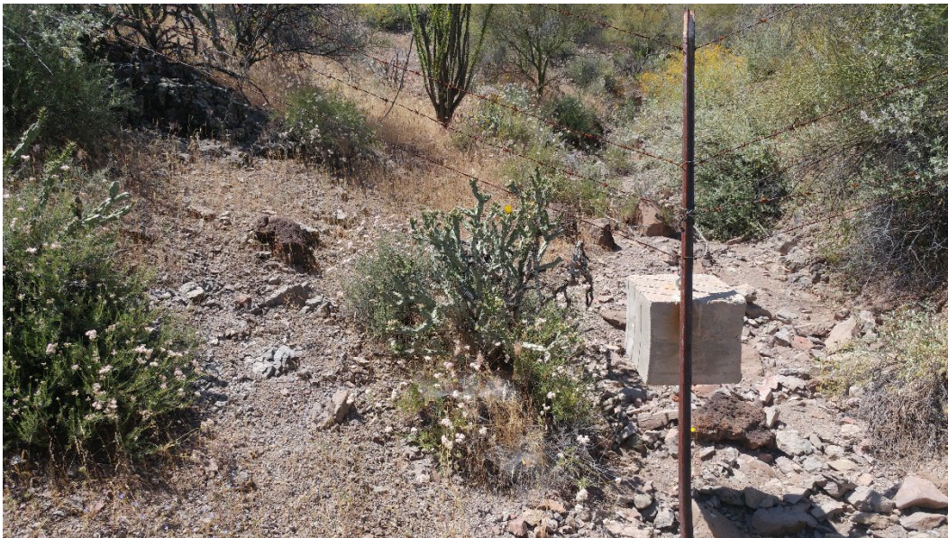
Figure 68. Deadweight Hang Anchoring a Fence Post Where ROW Fence Spans a Wash
