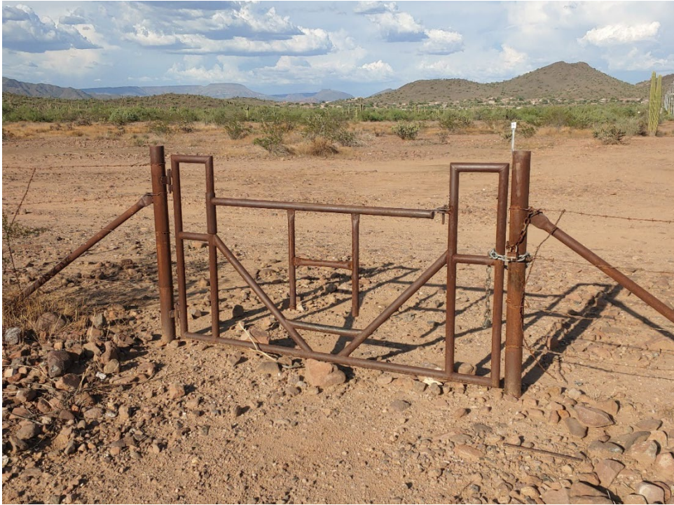
Figure 66. Modified Equestrian Gate to Prevent Burro Passage Through Aperture
