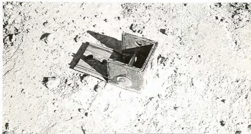
FIGURE A-55. SIGN INSTALLATION AFTER TEST 6. (BASE)
