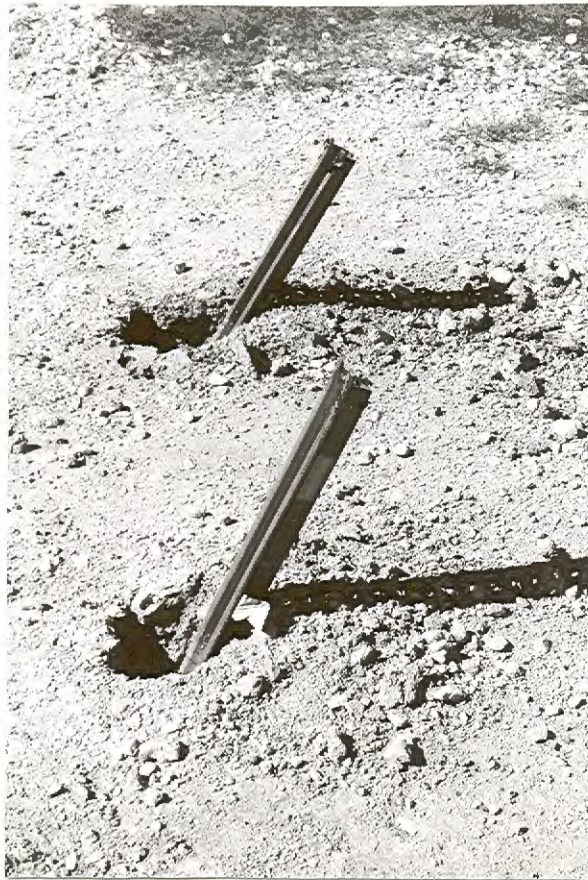
FIGURE A-85. SIGN INSTALLATION AFTER TEST 11.
