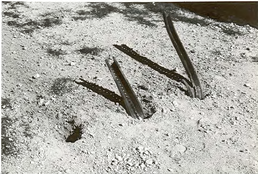
FIGURE A-117. SIGN INSTALLATION AFTER TEST 17.
