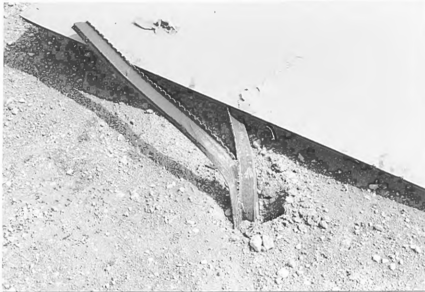
FIGURE A-147. SIGN INSTALLATION AFTER TEST 23.
