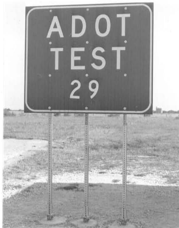
FIGURE 7.26. SIGN INSTALLATION USED IN TEST 7024-29.
