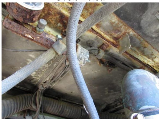
Top part of firewall on left side (close-up)
