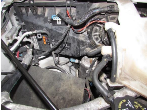
Left side of engine compartment – HVAC
