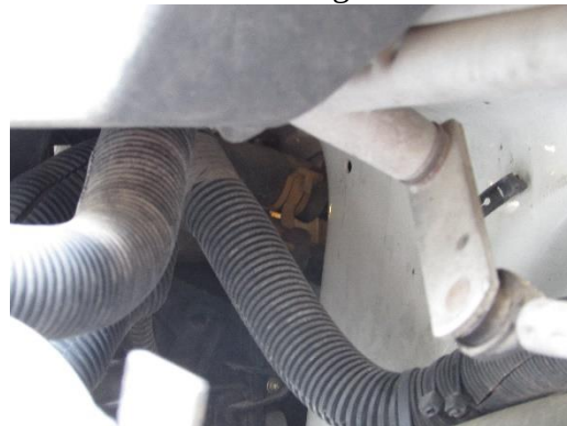
Penetrations on left side
