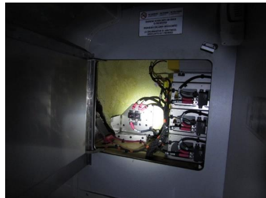
Cavity behind the lavatory mirror
