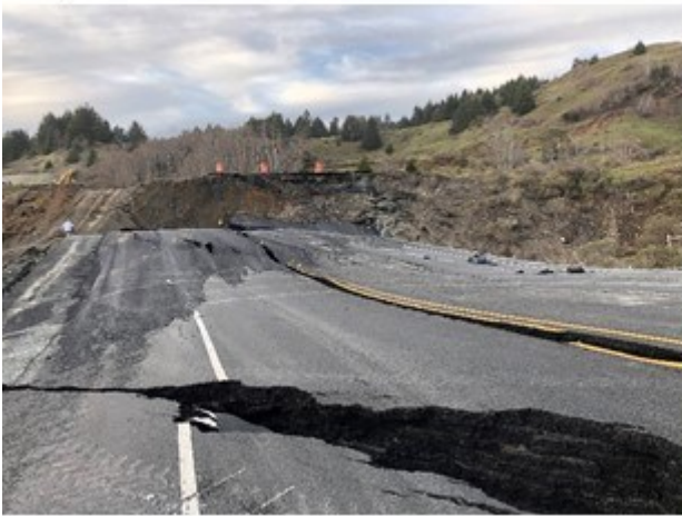
Figure 3.13: Photographs taken in early March 2019 shortly after the Hooskanaden landslide event. A). Shows uplift of the beach at the toe of the landslide. B). Shows an overview of the damage caused to HWY 101. C). Shows close up damage caused to the road by the landslide. D). Shows an example tension crack/scarp from the upper portion of the landslide (above the road).
