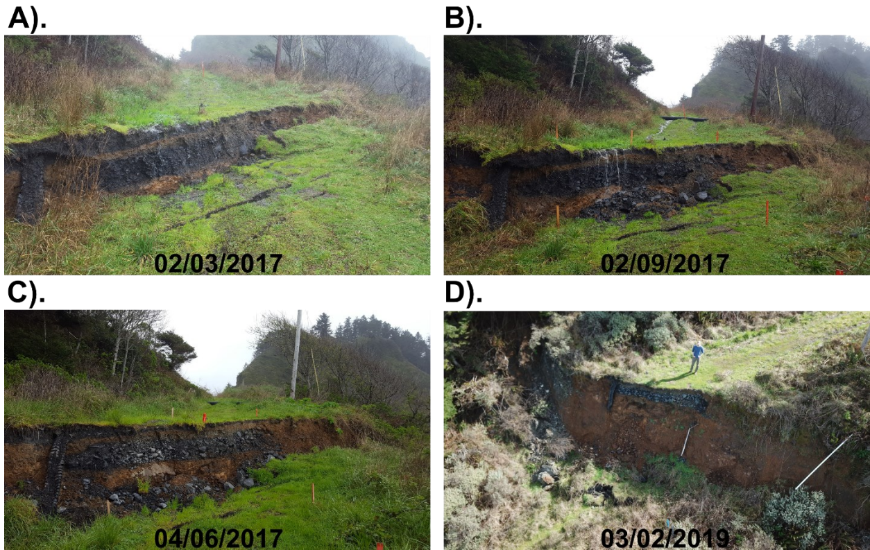
Figure 3.6: Development of a headscarp of a smaller progressive landslide within the main landslide body at Arizona Inn directly above the sea cliff from February 2017 (A) to March 2019 (D).
