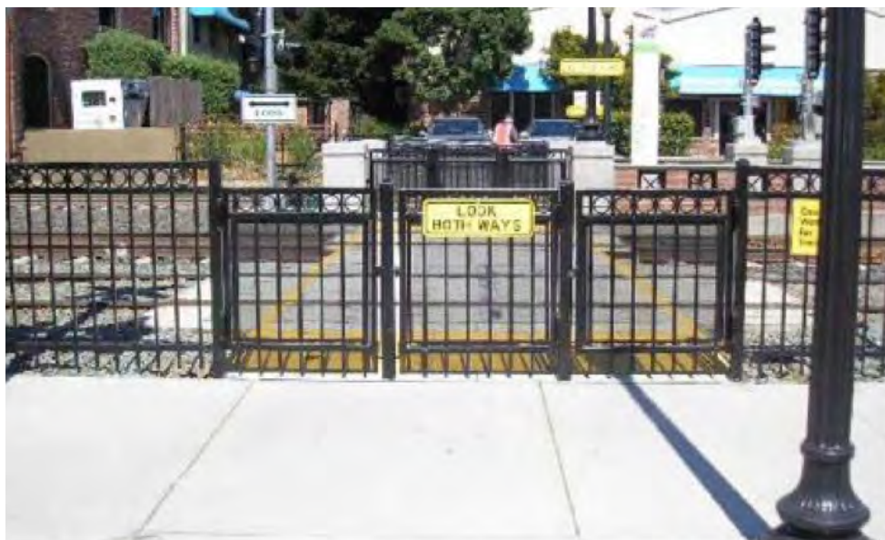
Figure 5-28 Pedestrian swing gate 23
