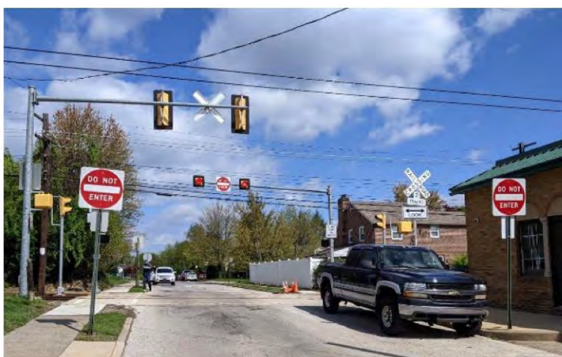
Figure 6-114 Variation on typical grade crossing for one-way street, looking against flow of traffic
