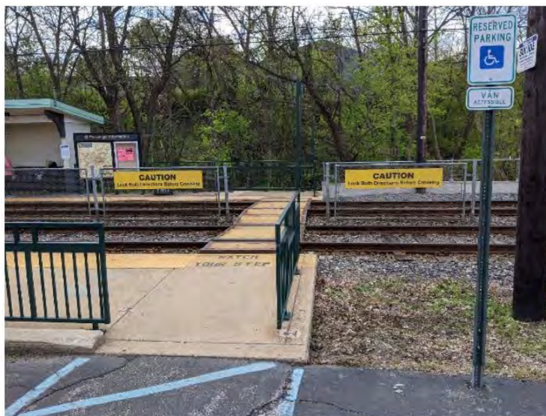
Figure 6-118 Pedestrian crossing at station on Media Line, not near street grade crossing
