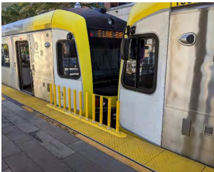
Figure 6-37 Station platform-edge bollards to prevent boarding between cars
