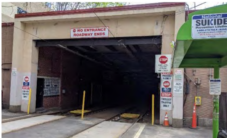
Figure 6-100 Signage at 36th Street Portal with signs for both motorists and SEPTA operators
