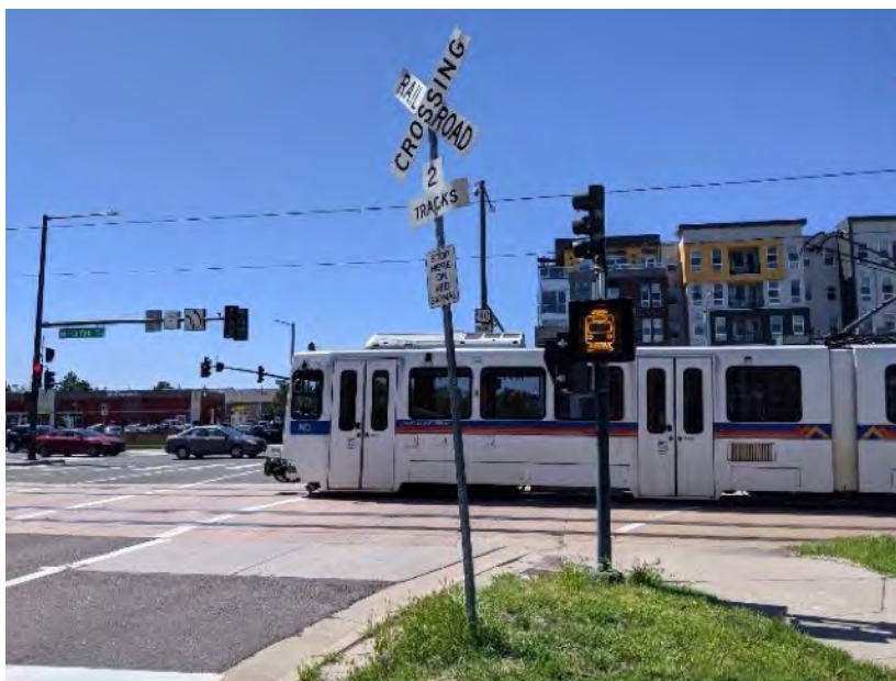
Figure 6-56 6-56 Crossbucks and dynamic signs at intersection near transition to dedicated right-of-way; note that dynamic signs alternate between “No Right Turn” and “Train” warning
