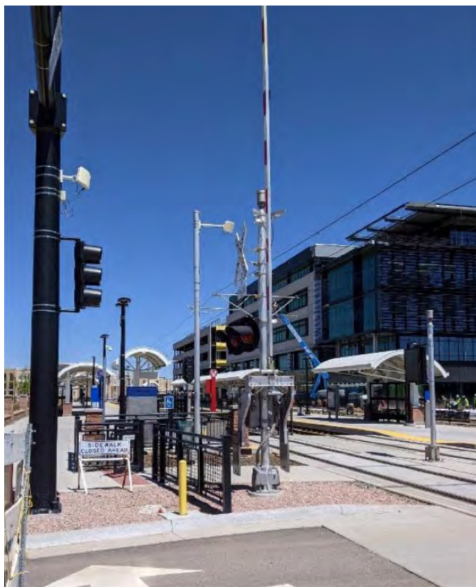
Figure 6-71 Grade Crossing at Sky Ridge Station; two sensors for occupancy detection system— one on traffic signal pole, one on its own pole
