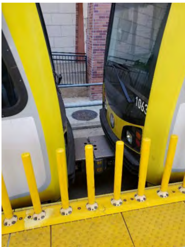
Figure 6-38 Station platform-edge bollards to prevent boarding between cars
