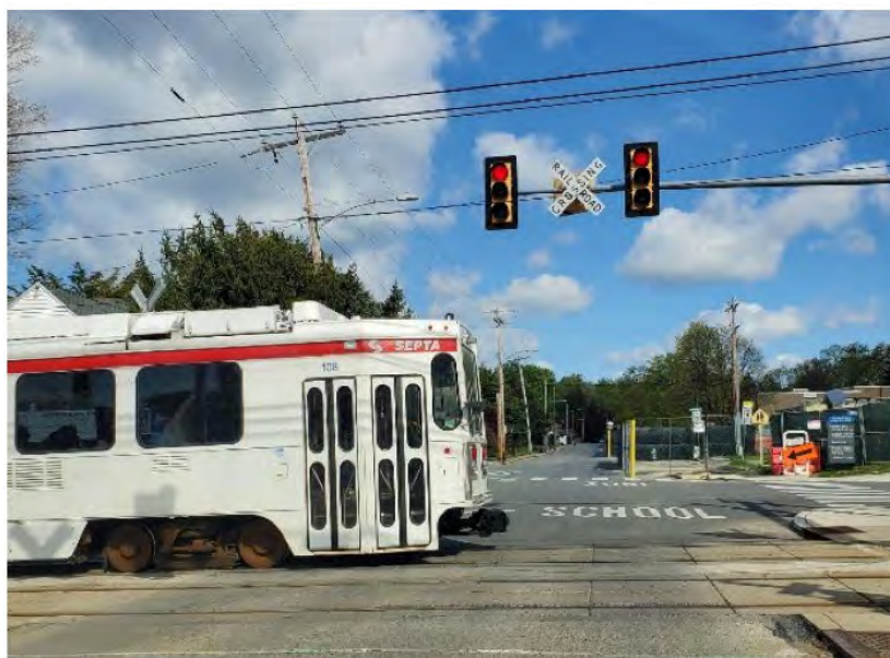
Figure 6-108 Detail of grade crossing traffic signals, high enough to be seen over train
