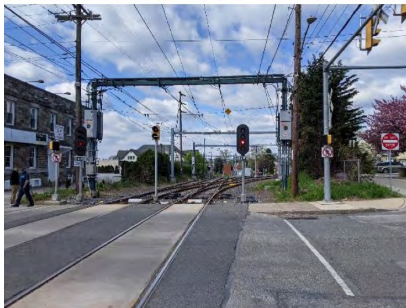
Figure 6-106 Color-light signals and bar signals at Drexel Hill Junction
