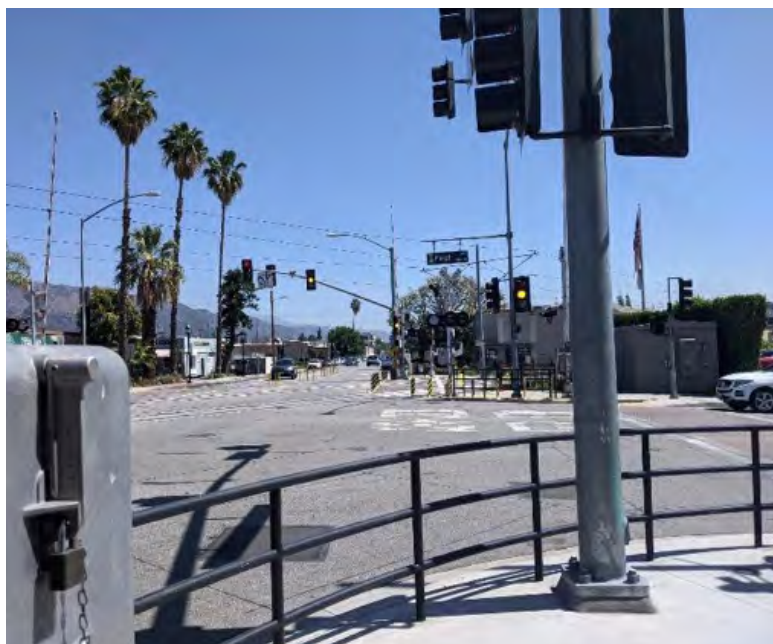
Figure 6-40 South corners of Arcadia intersection grade crossing showing pedestrian railing, bollards, crossbucks, flashers, gates
