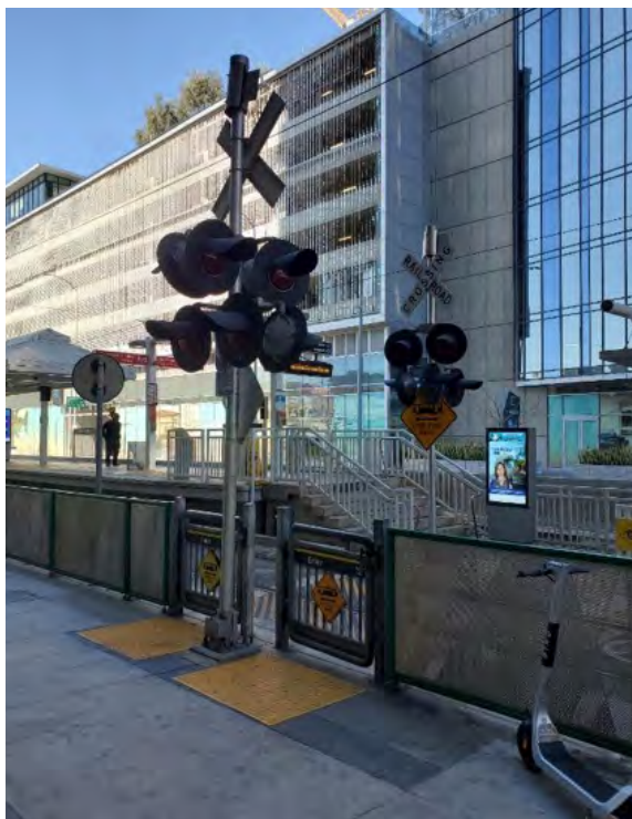
Figure 6-35 Pedestrian crossing at a station, protected by crossbucks, flashers, swing gates, pavement treatment, “Look Both Ways” warning signs
