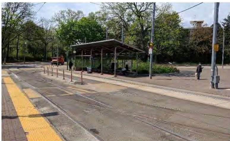
Figure 6-101 Pedestrian safety features at 40th Street Portal station
