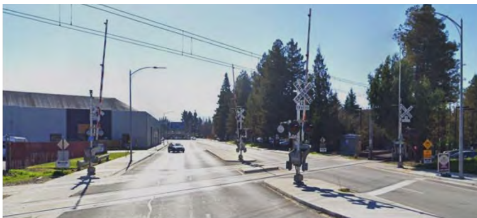
Figure 5-23 Pedestrian crossing with gates between roadway and sidewalk; no gate protection provided for pedestrians 19
