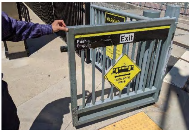
Figure 6-42 Signage on reverse side of one-way swing gate, marked as exit
