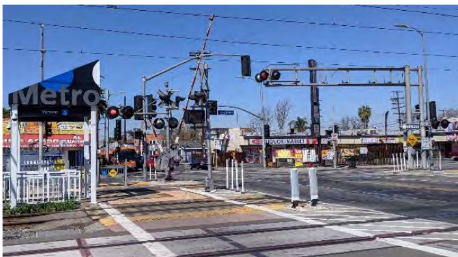
Figure 6-20 Use of bollards and pavement markings to provide separation at grade crossing
