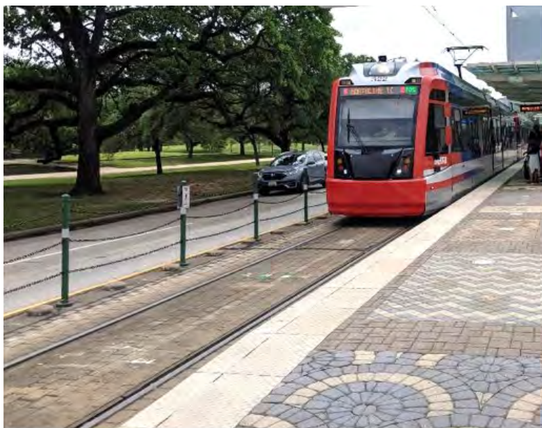
Figure 6-2 Houston Metro rail lane separation provided by brick pavement, concrete domes, fencing
