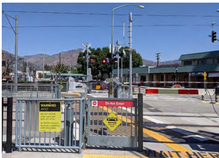
Figure 5-33 Warning signage on pedestrian crossing swing gates
