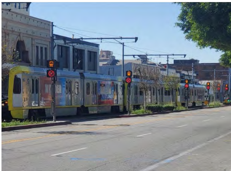
Figure 5-35 Motorist dynamic signage at private driveway entrances
