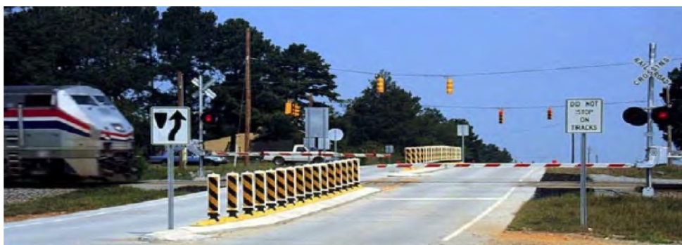
Figure 5-25 Concrete median divider with channelization devices 21
