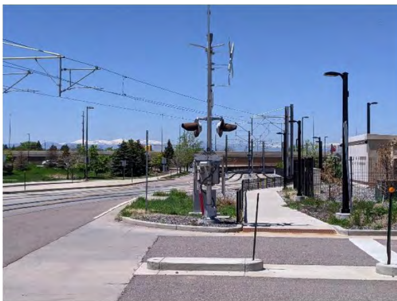
Figure 6-88 Grade crossing and track transition at northwest corner of R Line diversion, westward view showing track shifting to north
