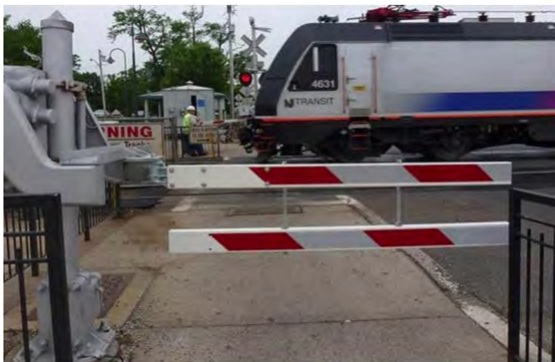
Figure 5-29 Pedestrian crossing gate with gate skirt 24
