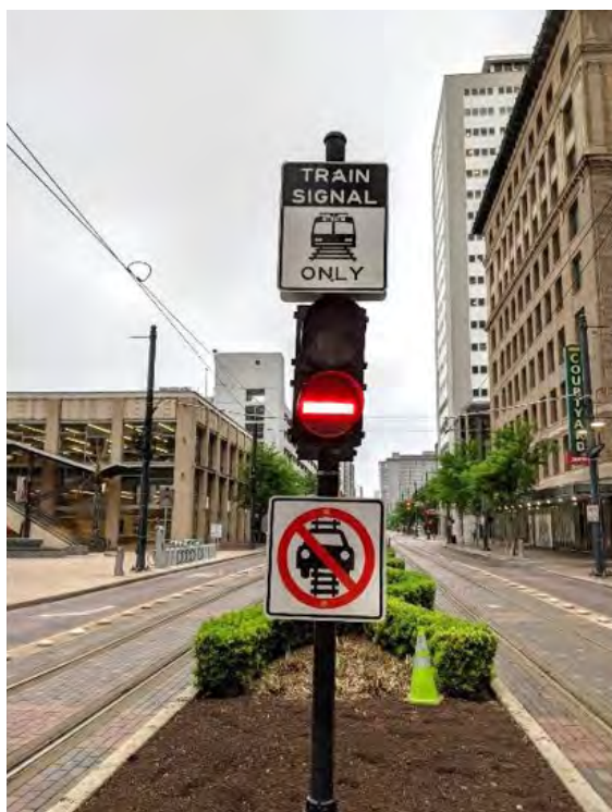
Figure 6-11 Red horizontal bar signal for train operation plus signage for motorists
