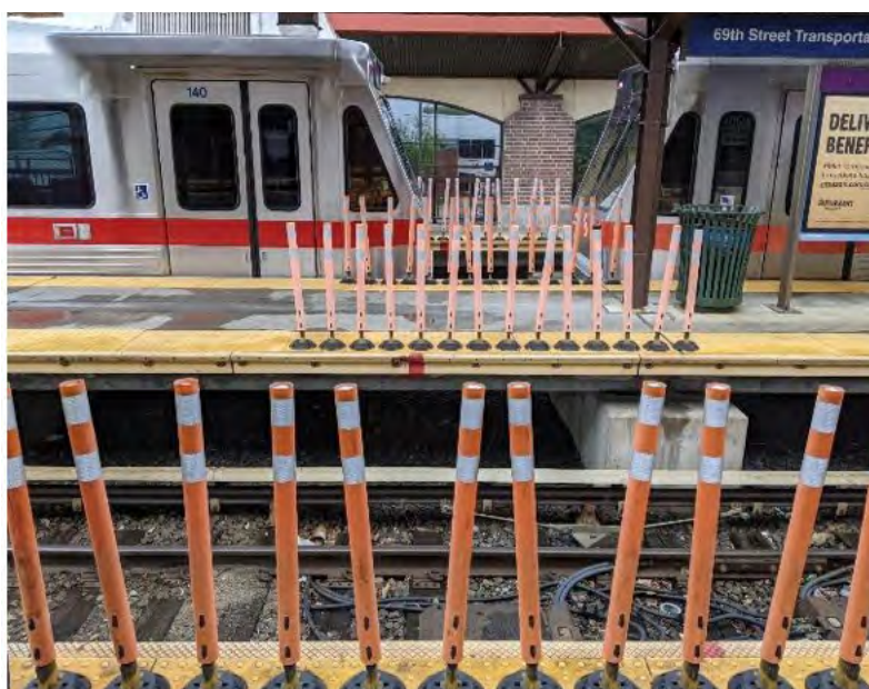
Figure 6-119 Bollards to prevent passengers from crossing between cars on high-level platforms for Norristown High Speed Line at 69th Street Transportation Center
