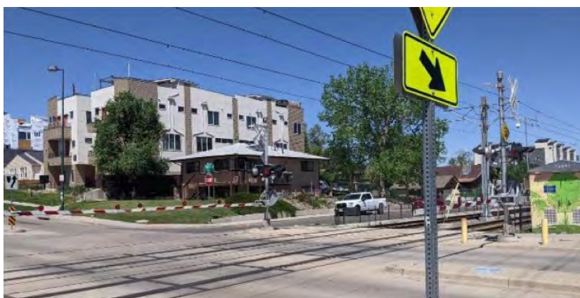
Figure 6-58 Typical crossing on West Line, looking northeast; three-quadrant gates down, intersect side street
