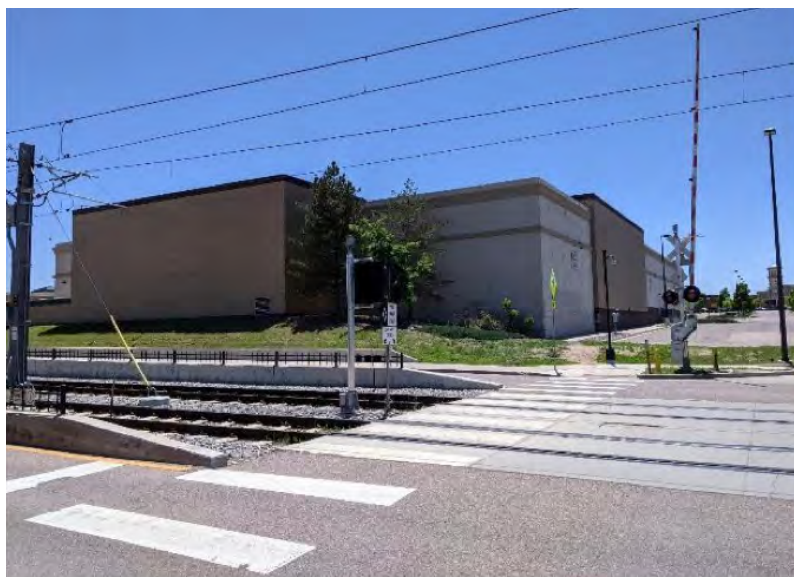
Figure 6-86 Grade crossing and track transition at northwest corner of R Line diversion, east side of intersection
