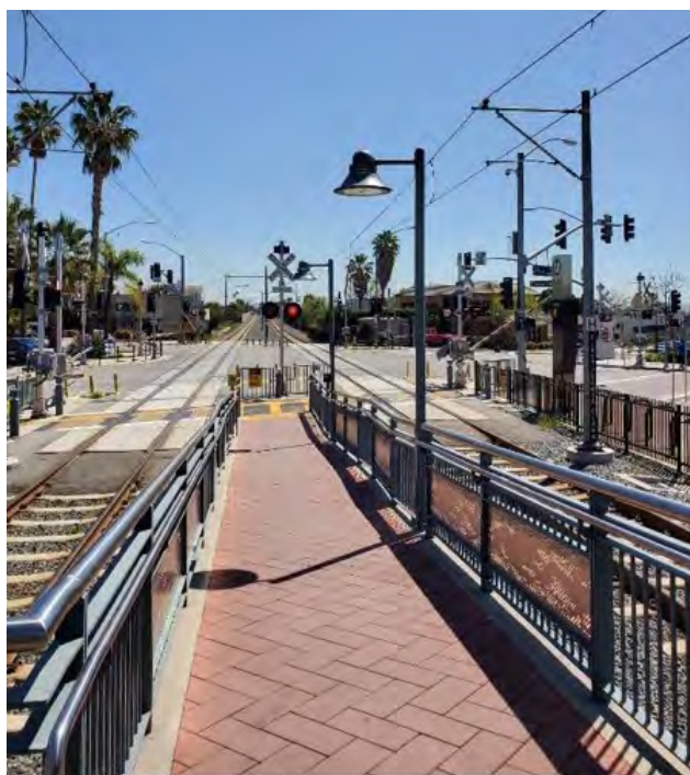
Figure 6-43 Arcadia intersection grade crossing from station platform, showing warning flashers and fencing
