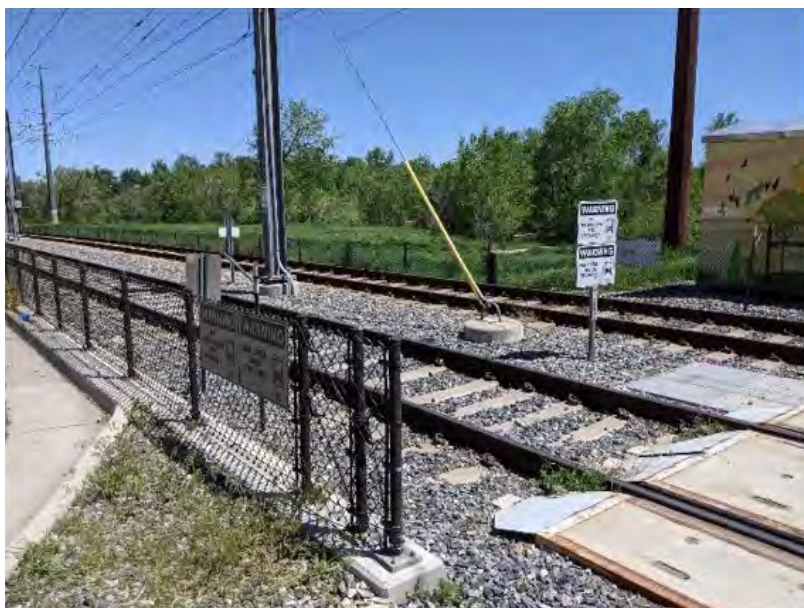
Figure 6-59 Typical crossing on West Line; signage and right-of-way fencing
