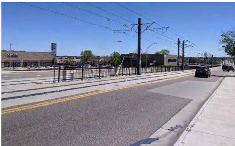
Figure 6-73 South portion of R Line diversion with embedded track, low curb, center fence
