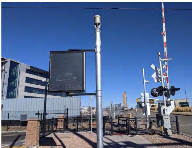
Figure 6-69 Grade Crossing at Sky Ridge Station; dynamic sign also has message for approach of second train
