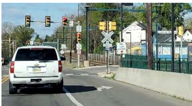
Figure 6-116 Grade crossing with separate traffic signal and signage for right turn across tracks
