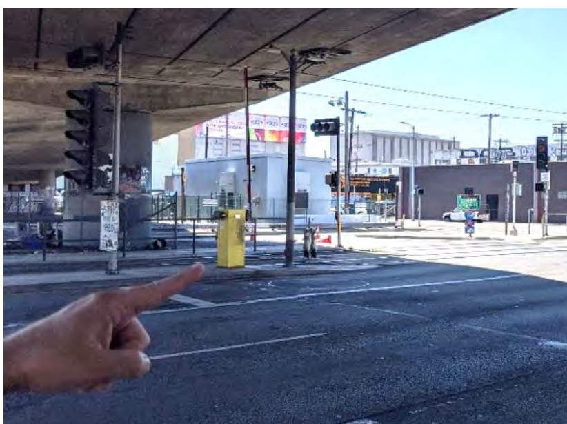
Figure 6-28 Use of parking lot style gate arm in street-running for left-turn lane with insufficient space for conventional gate arm mechanism
