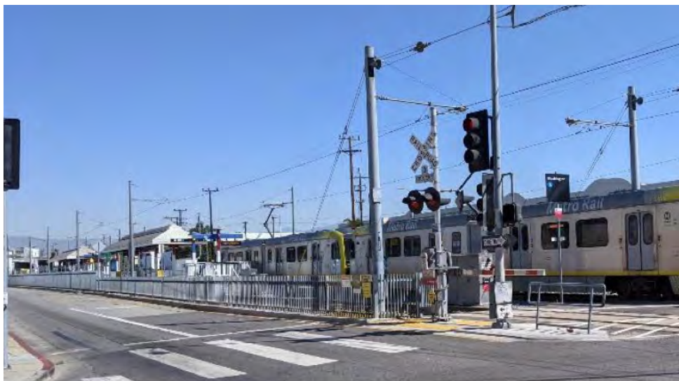
Figure 6-17 Fencing along A (Blue) Line; shorter fencing used near grade crossings to improve visibility
