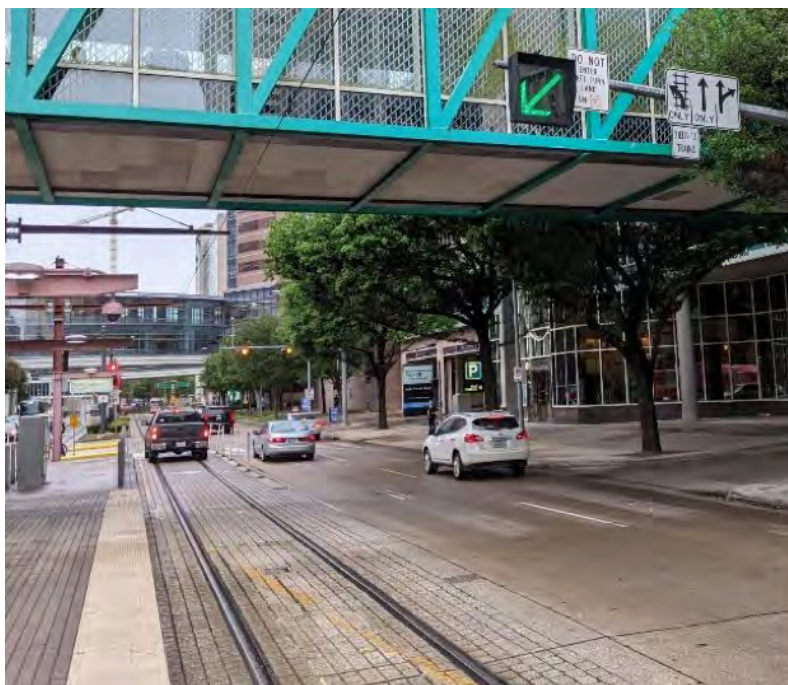
Figure 6-4 Rail lane shared as left-turn-only lane, including signage
