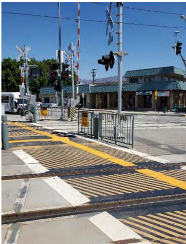
Figure 6-44 Detail of fencing, crossbuck, and flashers protecting detraining passengers
