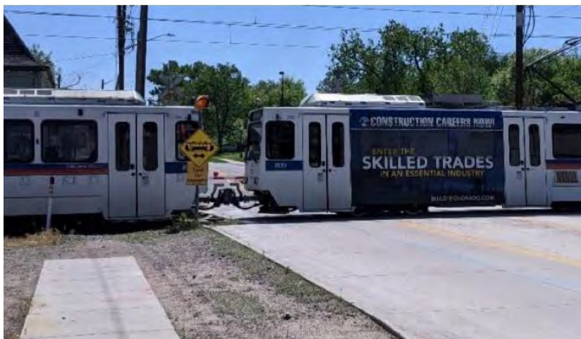
Figure 6-64 Supplemental warning signs and amber flashing light on left side of road for light rail tracks only at shared corridor crossing
