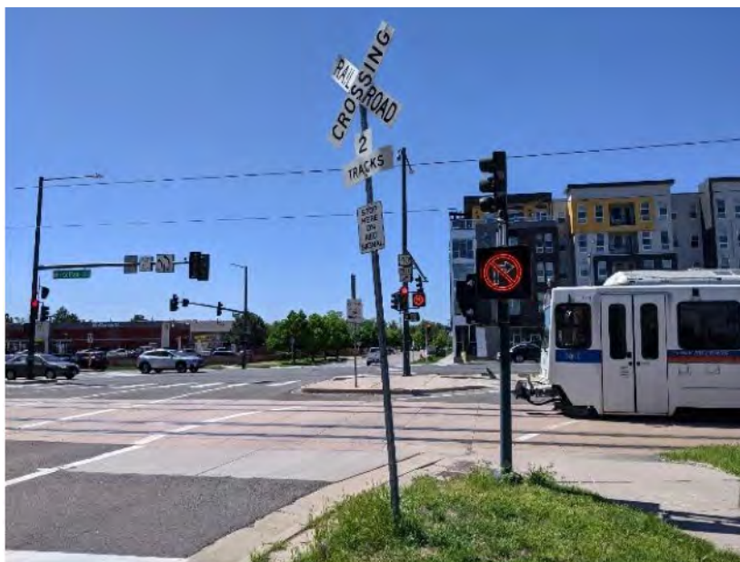
Figure 6-55 Crossbucks and dynamic signs at intersection near transition to dedicated right-of-way; dynamic signs alternate between “No Right Turn” and “Train” warning
