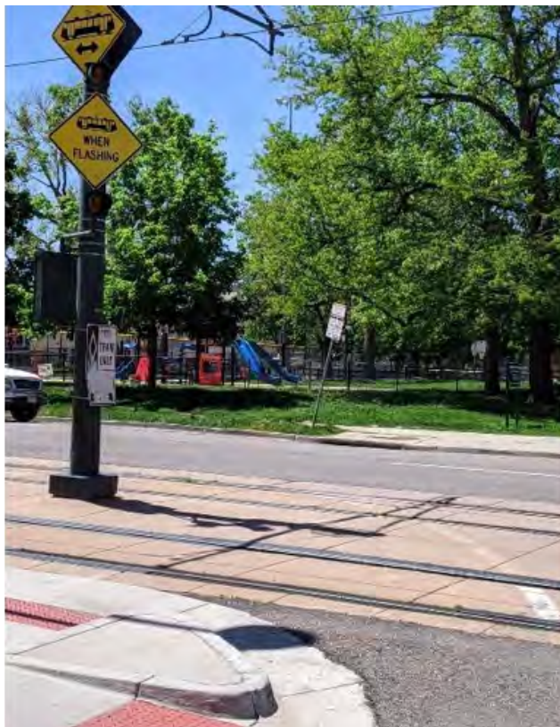
Figure 6-52 Additional warning signage and flashing amber lights at intersection on L Line
