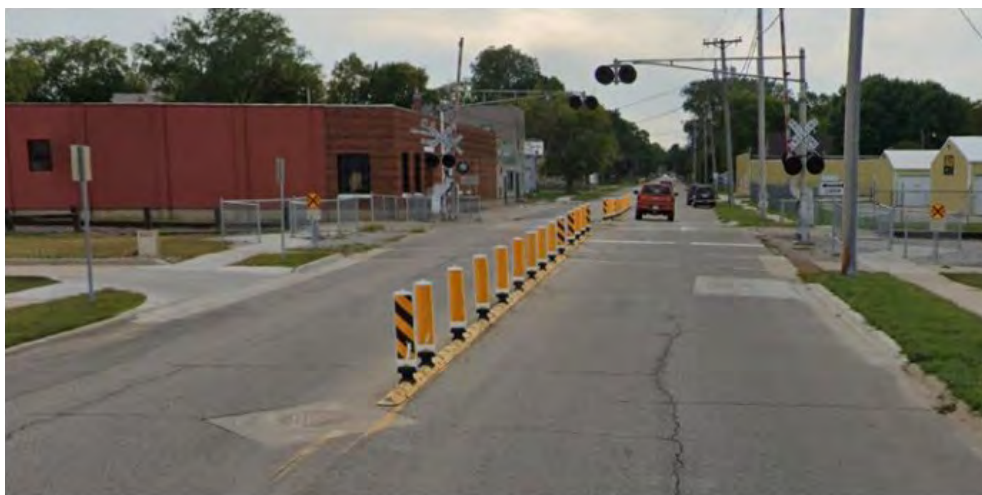
Figure 5-26 Channelization devices 22
