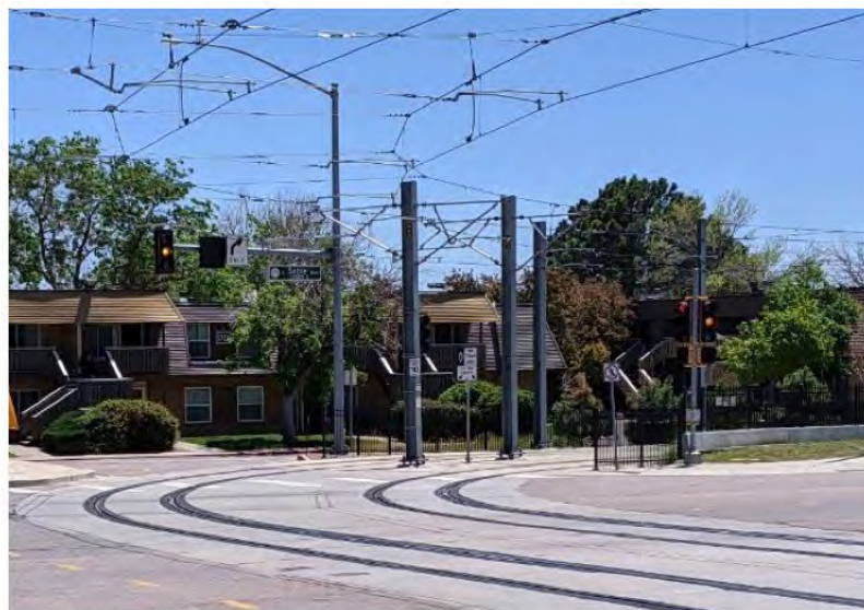
Figure 6-83 Closer view of transition and signage on east side of intersection
