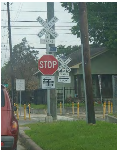
Figure 6-15 Crossbuck protection at minor side-street grade crossing
