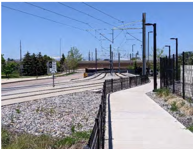
Figure 6-89 Grade crossing and track transition at northwest corner of R Line diversion, westward view showing west end and final track transition; pavement marking and sign to discourage motorists from entering transit right-of-way
