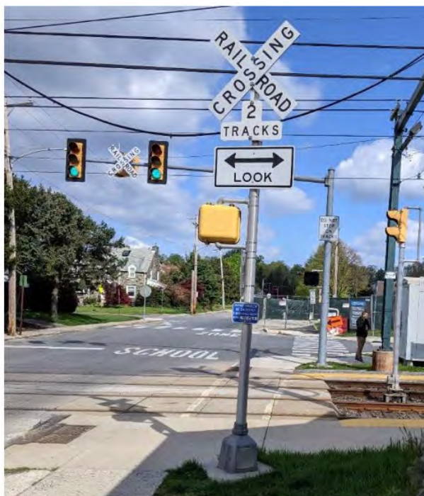
Figure 6-109 Detail of pedestrian crossing signals, pavement markings, signage
