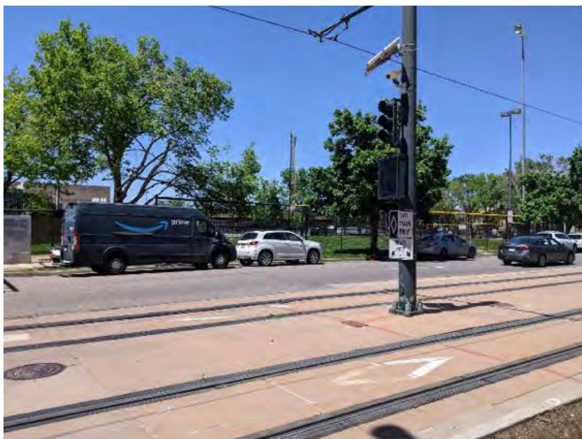
Figure 6-50 L Line street-running two-track section; note signage, pavement markings, location of catenary pole between tracks
