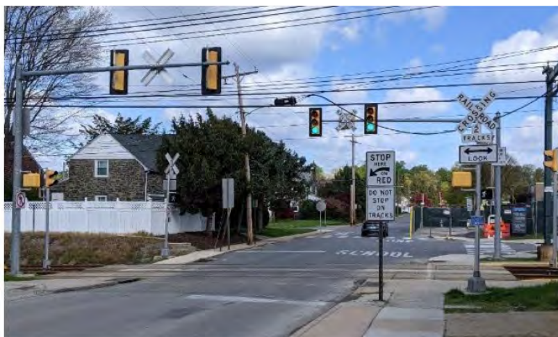
Figure 6-107 Overall view of typical grade crossing on Routes 101 and 102 with crossbucks, traffic signals including pedestrian signals, additional signage and pavement markings, bar signals for trains
