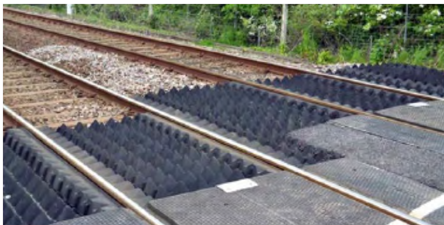
Figure 5-31 Anti-trespass panels 26
