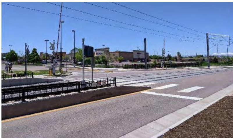
Figure 6-85 Grade crossing and track transition at northwest corner of R Line diversion; conventional grade crossing flashing lights, bells, gates, raised medians, dynamic sign for pedestrians in use
