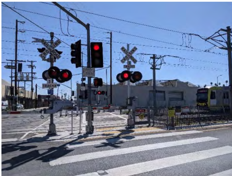
Figure 6-31 Grade crossing with additional pedestrian safety features, including flashers and gates, one-way swing gate, signage, pavement markings
