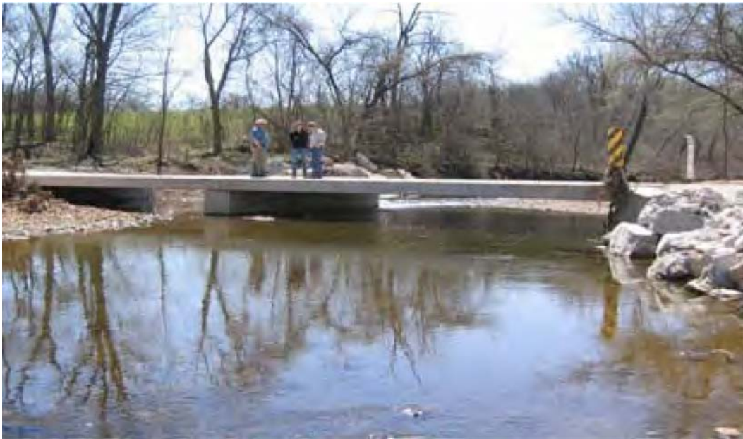
Figure 4. Low-water bridge (39).
