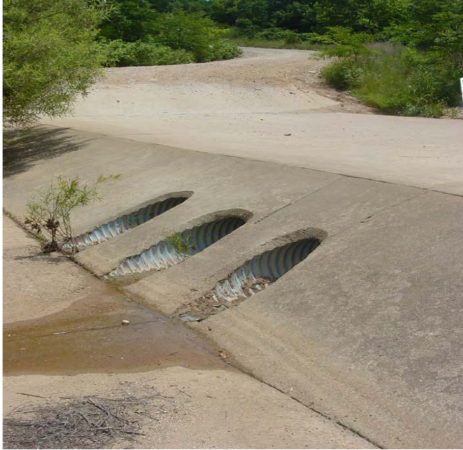
Figure 3. Vented low-water crossing (39).
