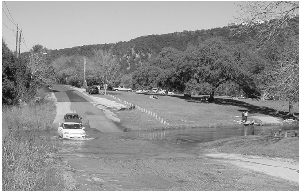
Figure 2. Unvented low-water crossing (38).
