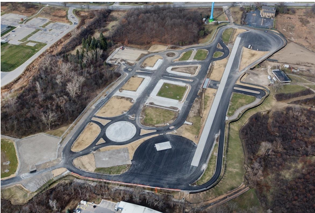
Figure 3: Aerial photo of Mcity under construction, Spring 2015.
