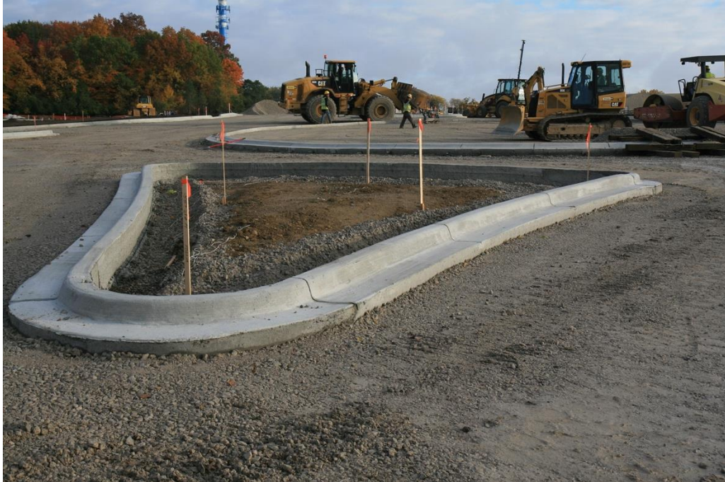
Figure 2: Roundabout under construction, Fall 2014.
