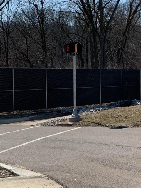
Figure 19: Pedestal-mounted pedestrian crossing signal.
