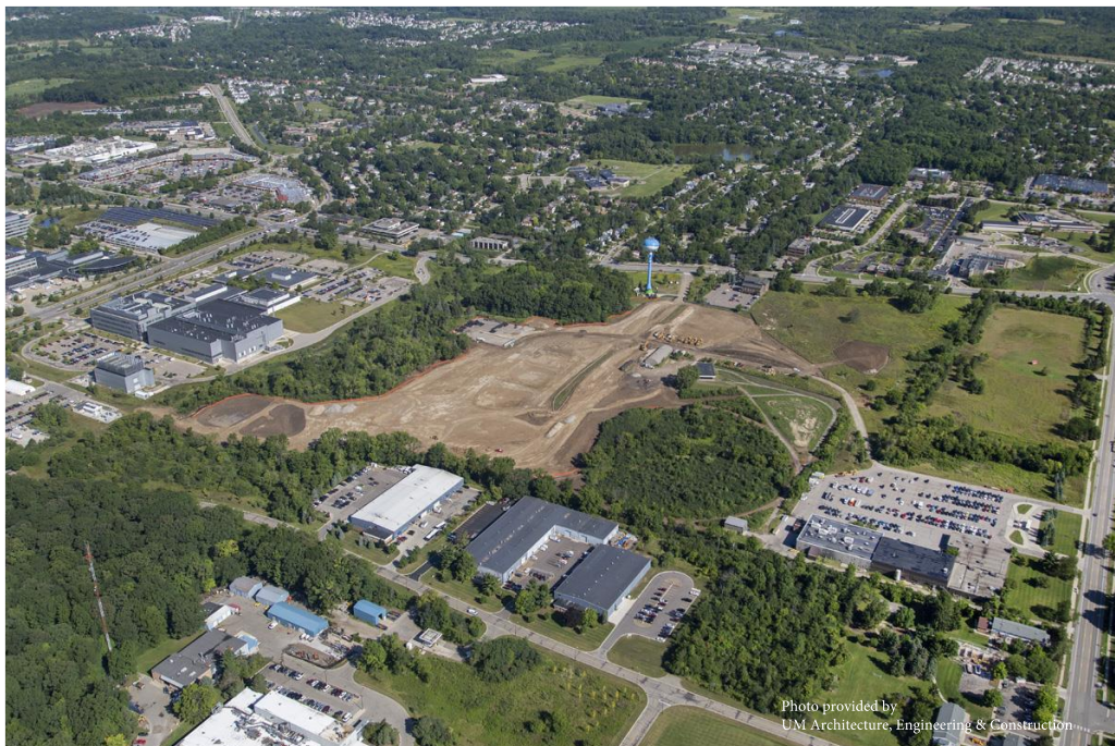
Figure 1: Aerial photo of Mcity under construction, Summer 2014.
