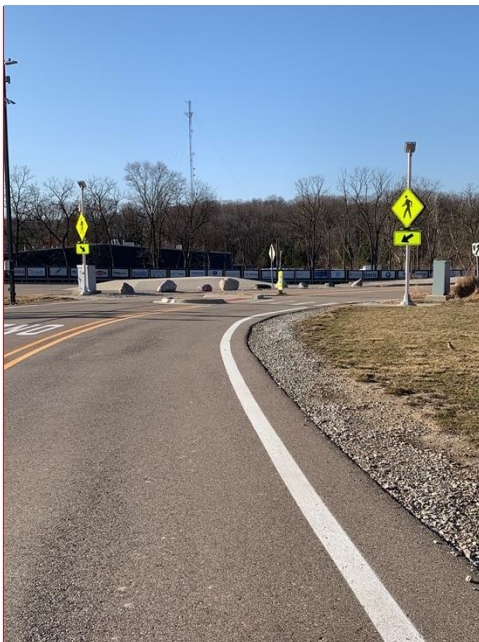
Figure 17: Mid-block pedestrian crossing with rapid RRFB.
