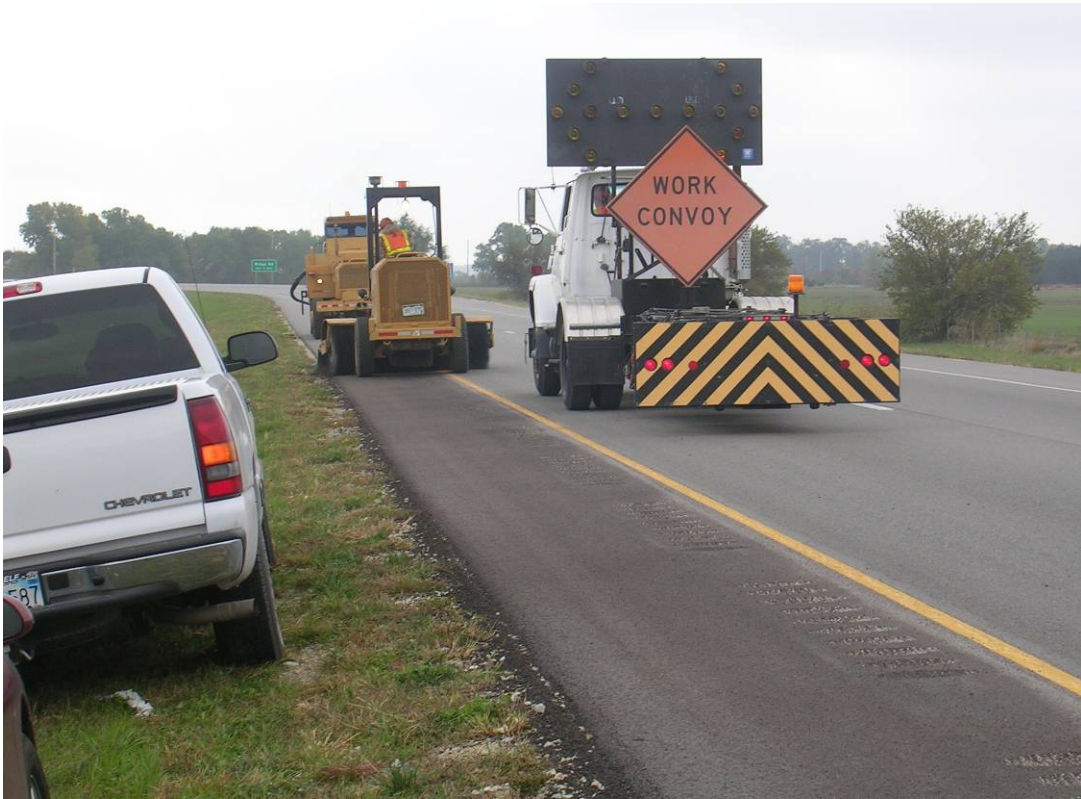
Figure A8: Work convoy cutting football shaped rumble strips and clearing debris
