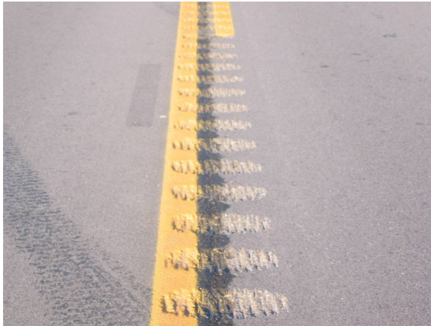
Figure 4.22: Centerline football shaped rumble strips along US Highway 40 (viewed parallel to the path of travel)
