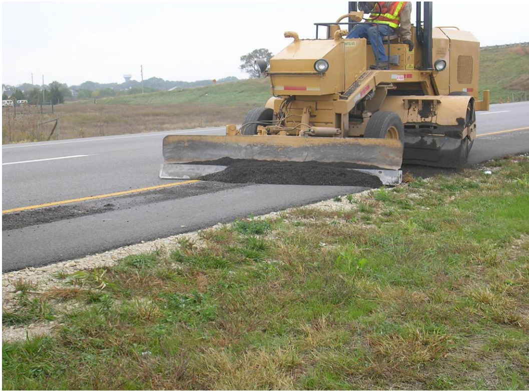
Figure A6: Cleaning apparatus following milling apparatus (Dustrol, Inc.)
