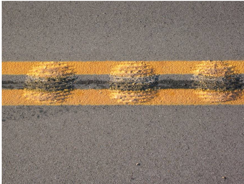
Figure 4.23: Centerline football shaped rumble strips along US Highway 40 (viewed perpendicular to path of travel)
