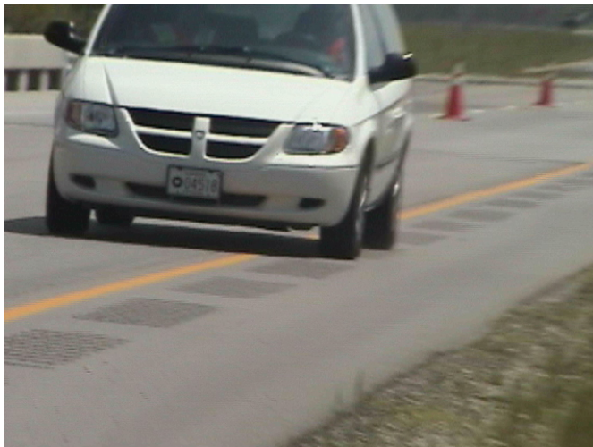
Figure 4.13: 2002 Dodge Caravan crossing rectangular rumble strips
