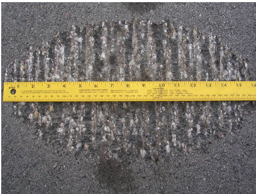
Figure A2: Length of single football shaped rumble strip (16 in.)
