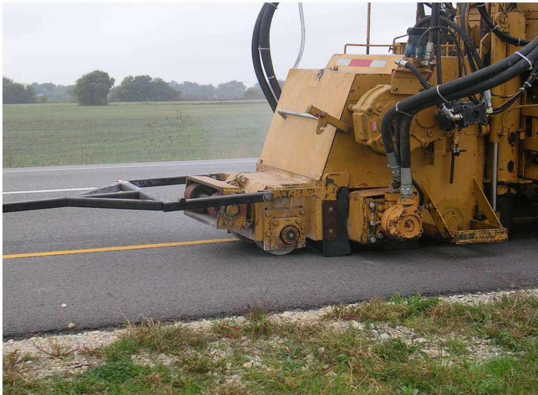
Figure A5: Milling apparatus for cutting football shaped rumble strips (Dustrol, Inc.)
