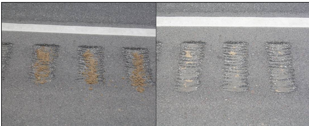
Figure 4.3: Rectangular Rumble Strips, Debris Test Trial 2 at time = 0 hr. (left) and at time = 18 hrs. (right).
