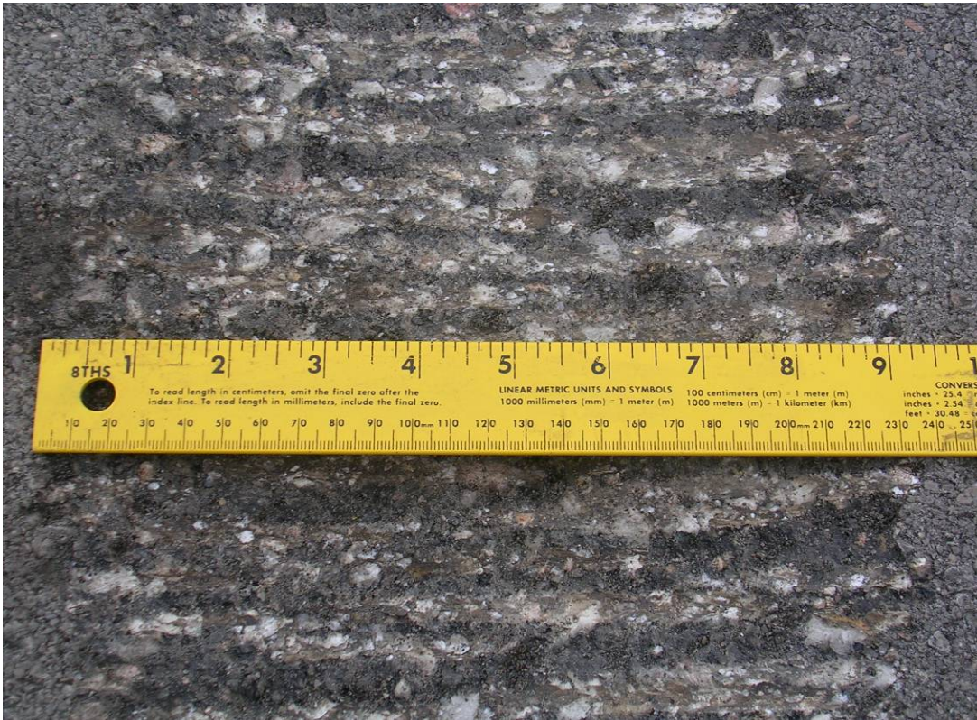
Figure A1: Width of single football shaped rumble strip (9 in.)
