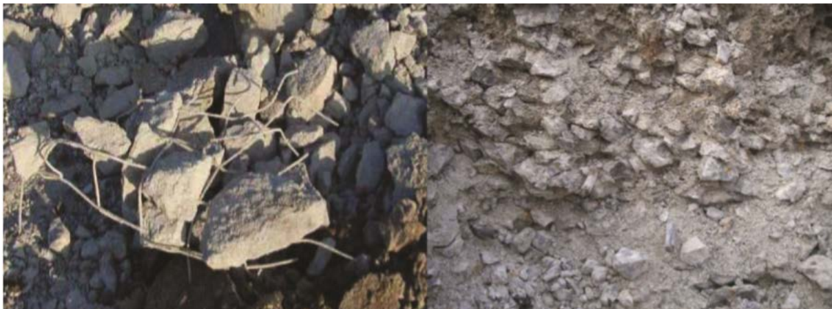
Figure 7. Rubblization size and depth: (a) Particle size viewed from the surface and (b) Influence depth seen from the side (28).
