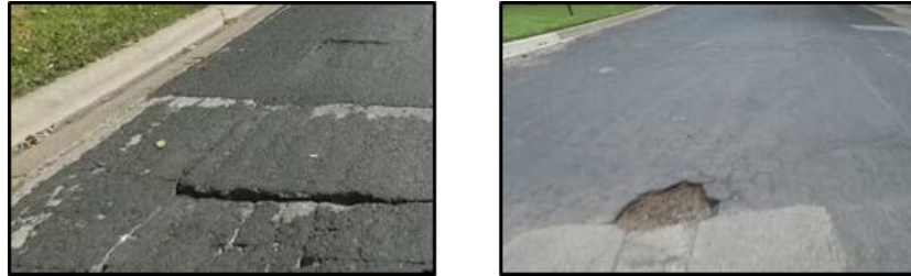
Figure 12. Instances of road damages: Deep transverse crack and pothole.
