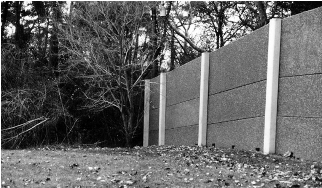
Figure 5. Example of Post-and-Panel System Using Concrete Posts (4).
