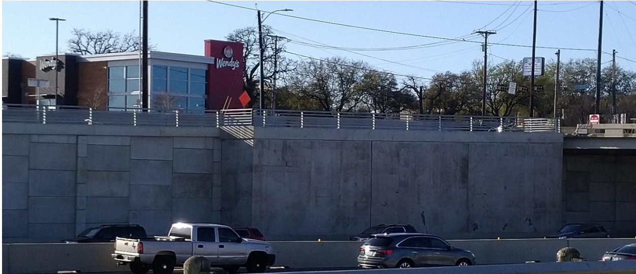
Figure 100. Retaining Wall B30C, Drilled Shaft Portion.
