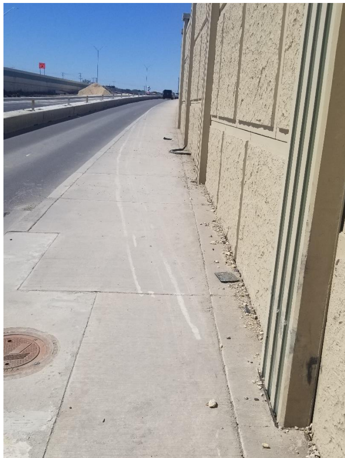
Figure 153. Visible Markings on SWNB04 and Sidewalk from Vehicle Strike.
