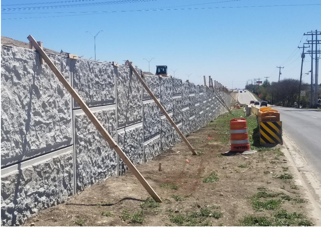
Figure 164. Temporary Construction Bracing at Face of RWSB01.
