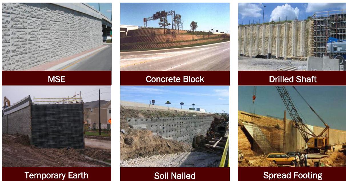
Figure 3. Types of Retaining Walls (15).
