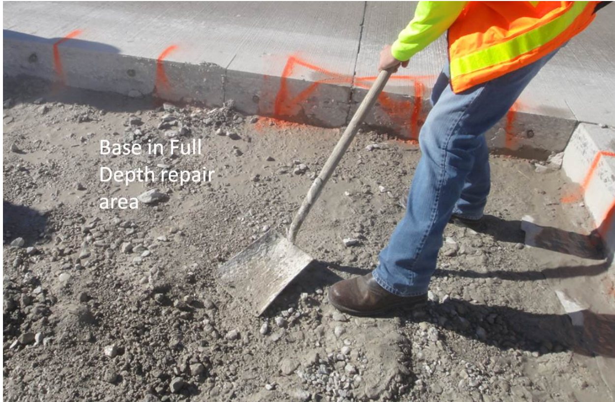
Figure 14. Existing Base on US 75 (Good Quality).
