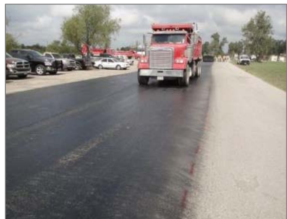
FIGURE 2 – Emulsion Trackless Tack Coat.
