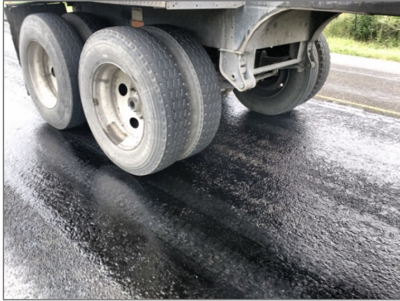
FIGURE 3 – Hot-Applied Trackless Tack Coat.
