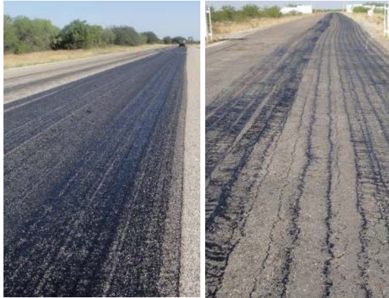
FIGURE 7 – Proper and Improper Application.
