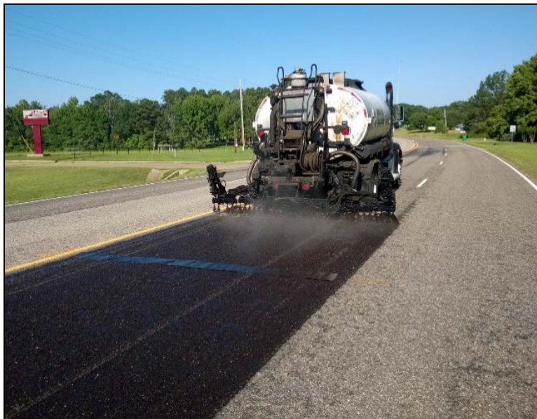
Figure 2-1. Traditional Tack Coat.
