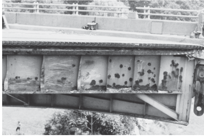
Figure 2.2. Collapse of the Mianus River Bridge (Fisher 1997).
