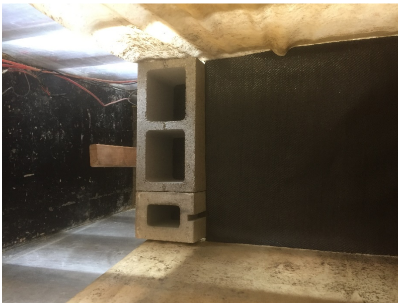
Figure 41. Compacting Backfill soil layer by layer
