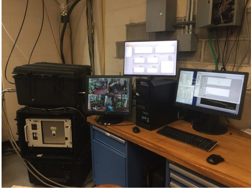
Figure 4: CEMS equipment integrated into the medium speed engine lab monitoring and control system.
